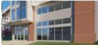
2 - BLD. 1 - RESIDENTIAL LOBBY ENTRANCE
