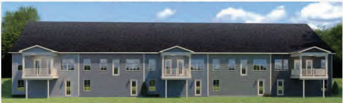
Walkout Basement Condition
