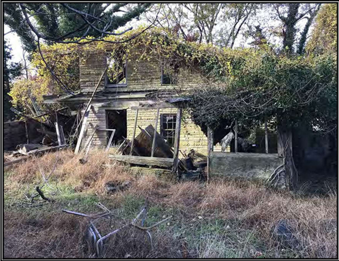
Figure 4-8. Photograph Depicting the Rear Side of the 1851 Butler House (Structure 2) [facing west]
