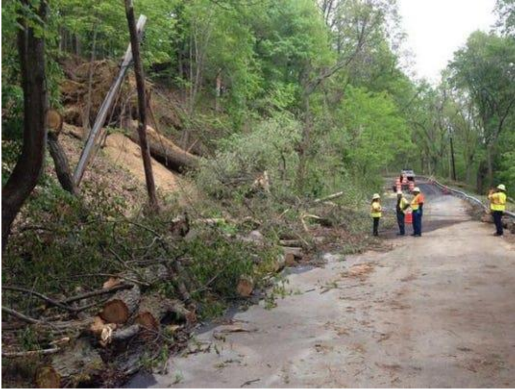
Figure 83. May 2014 Landslide in the Piscataway Hills community of Fort Washington
