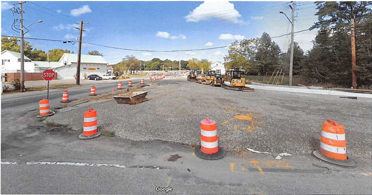
Intersection of Dyson Road and Brandywine Road looking west
