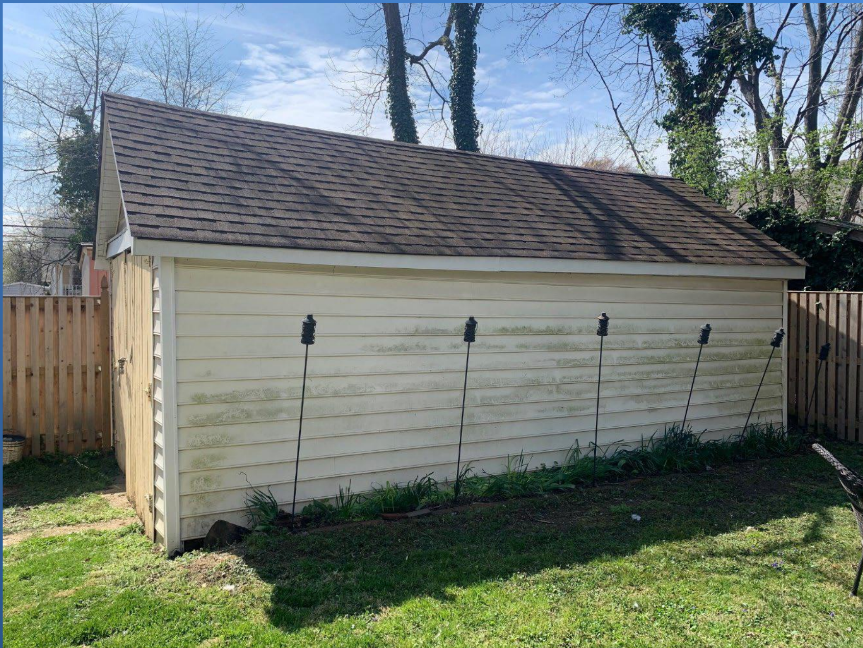
John and Mary White House, detached garage north elevation, April 2022
