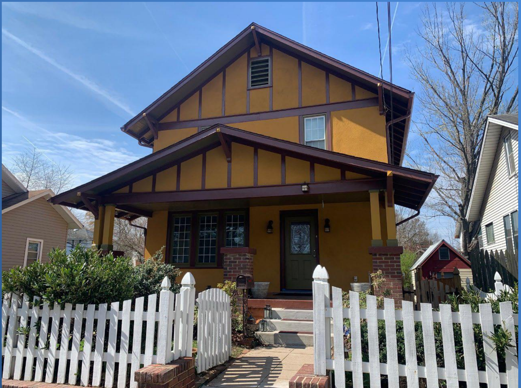
John and Mary White House, east elevation, April 2022
