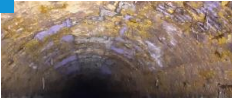
102" Anacostia Sewer Main Corrosion
