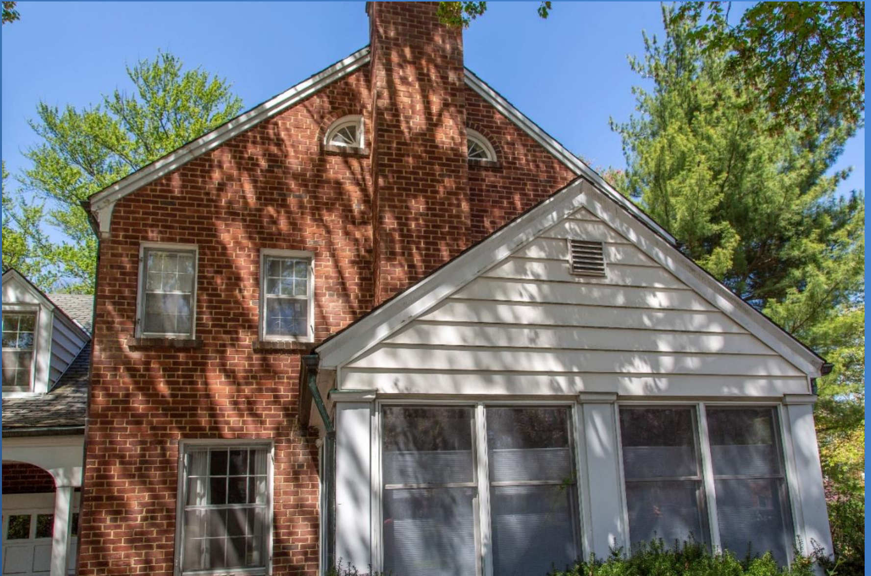
Boswell House partial south elevation, April 2023.
