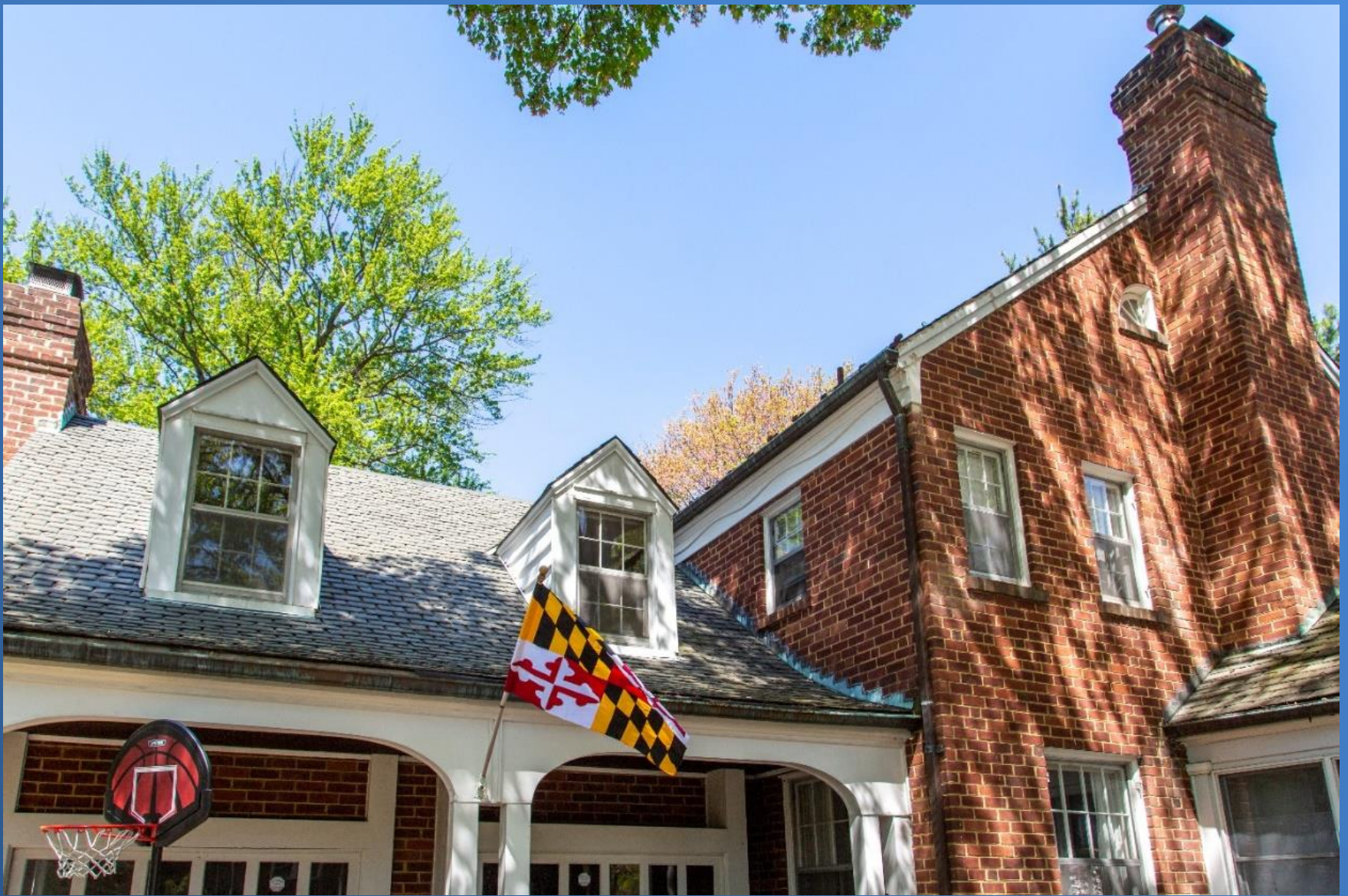
Boswell House partial south elevation, April 2023.
