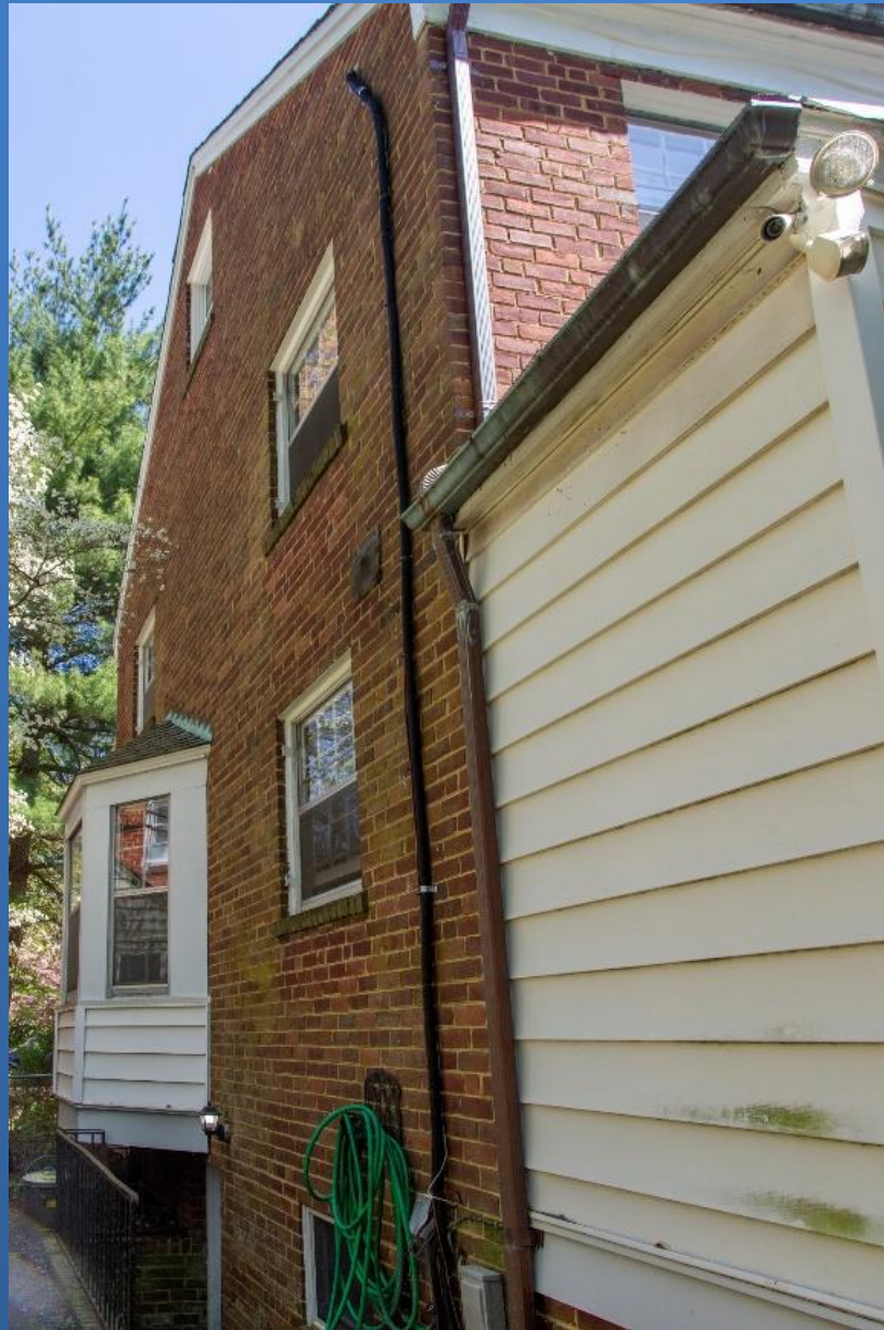
Partial north elevation, April 2023.
