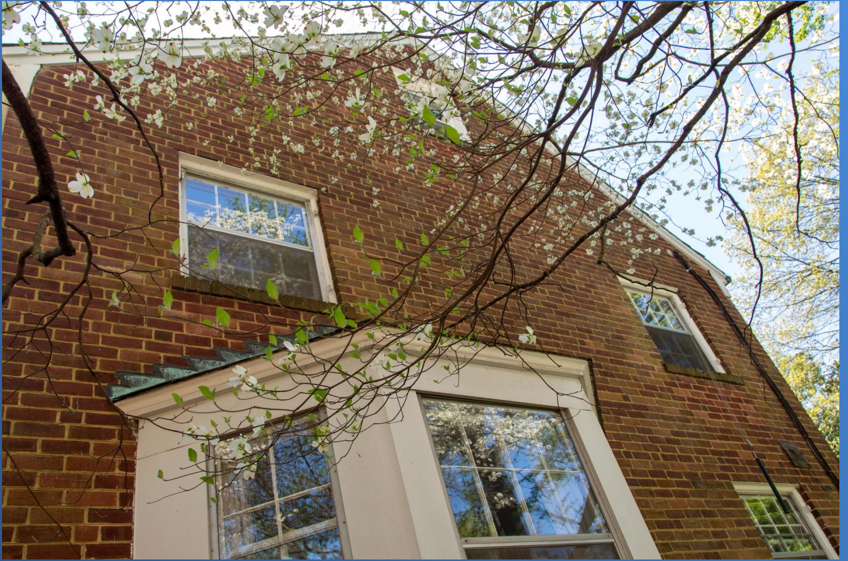
Partial north elevation showing fenestration of the main block, April 2023.
