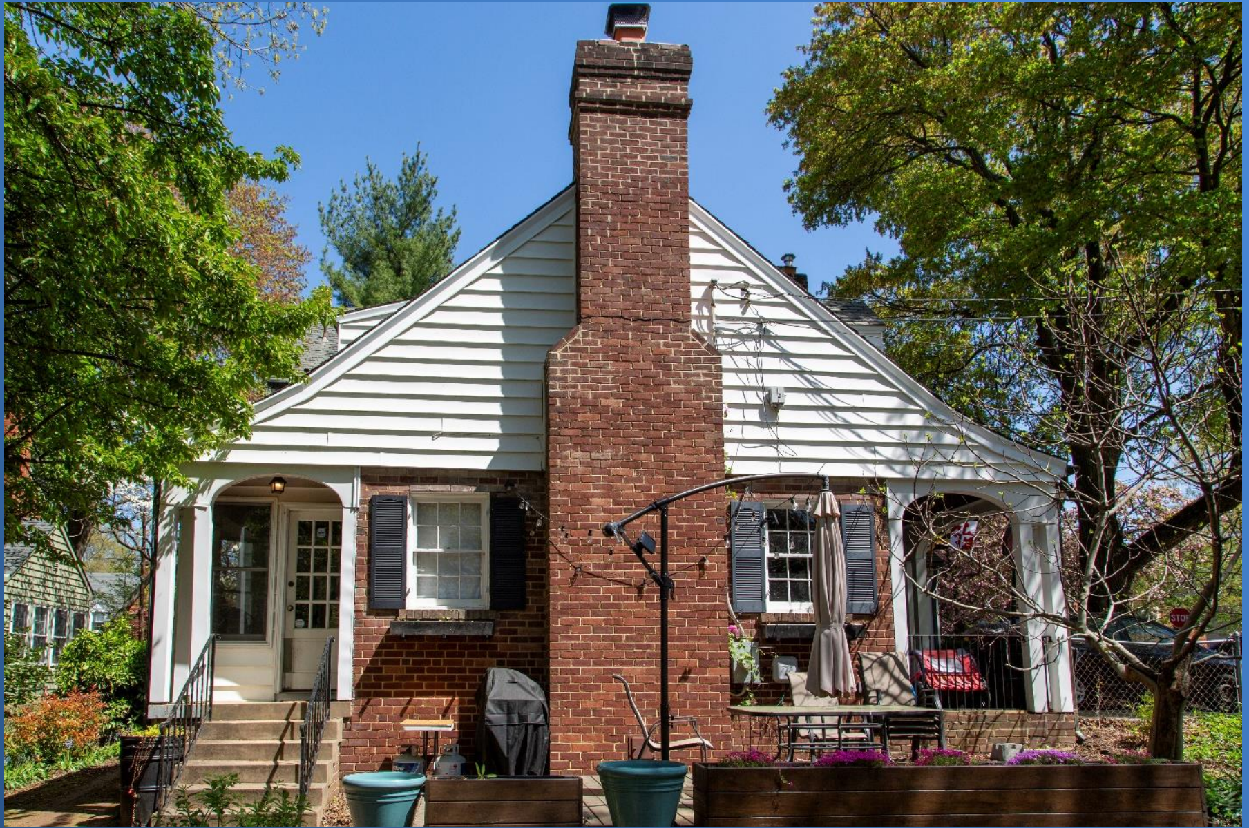
West (rear) elevation, April 2023.
