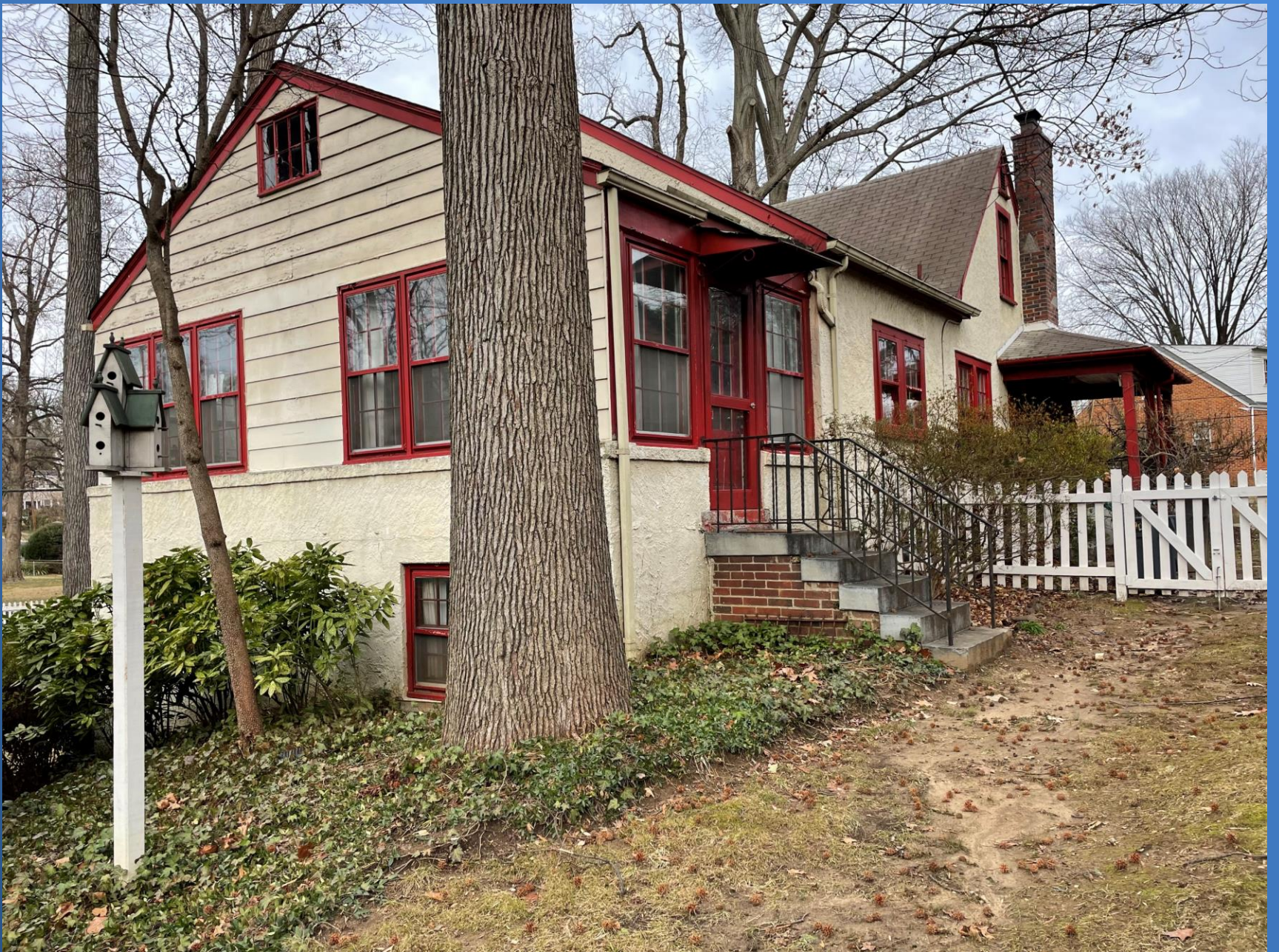
Blair-Smith House, southwest corner, January 2024.
