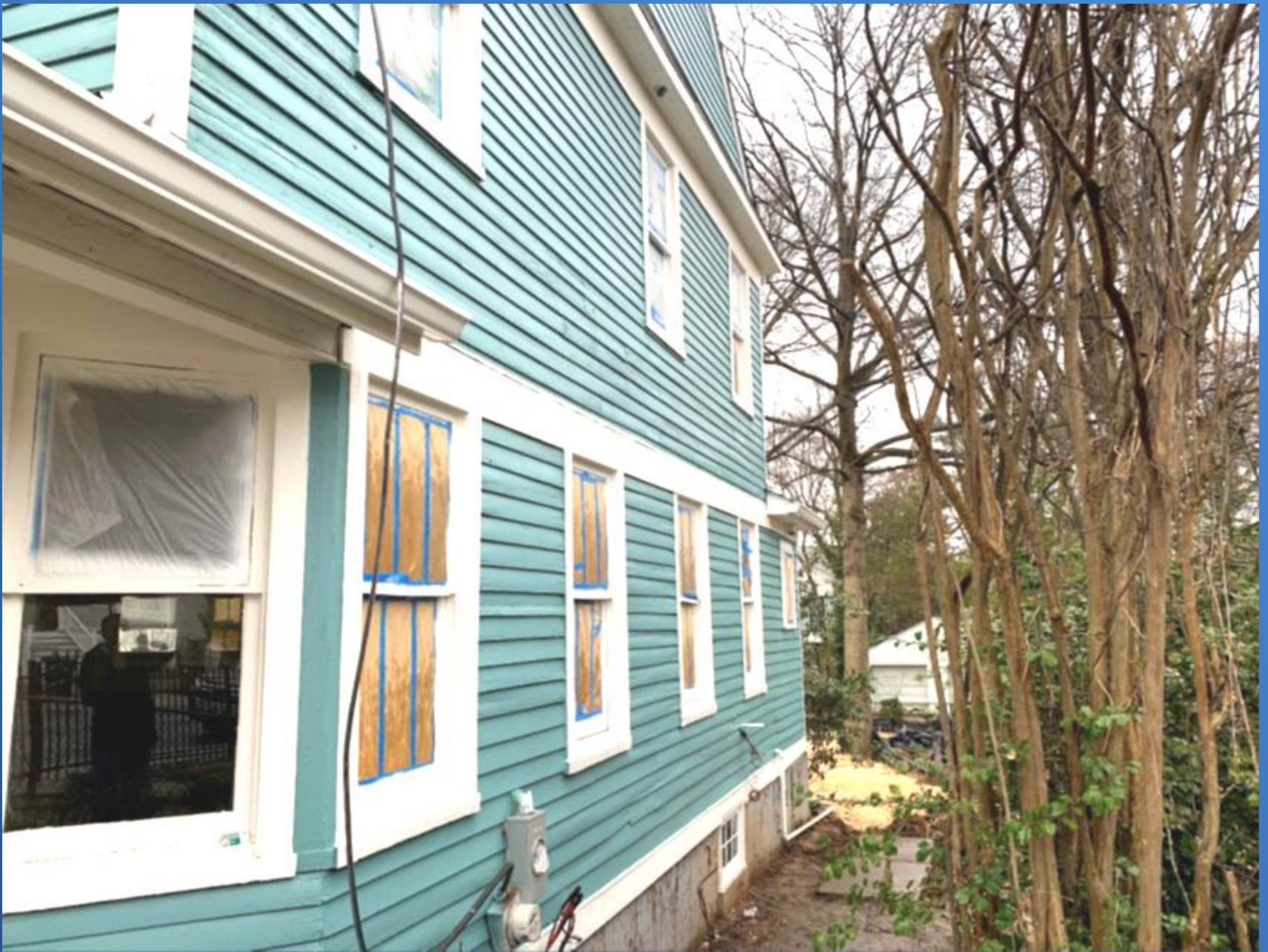
South elevation, February 2024.
