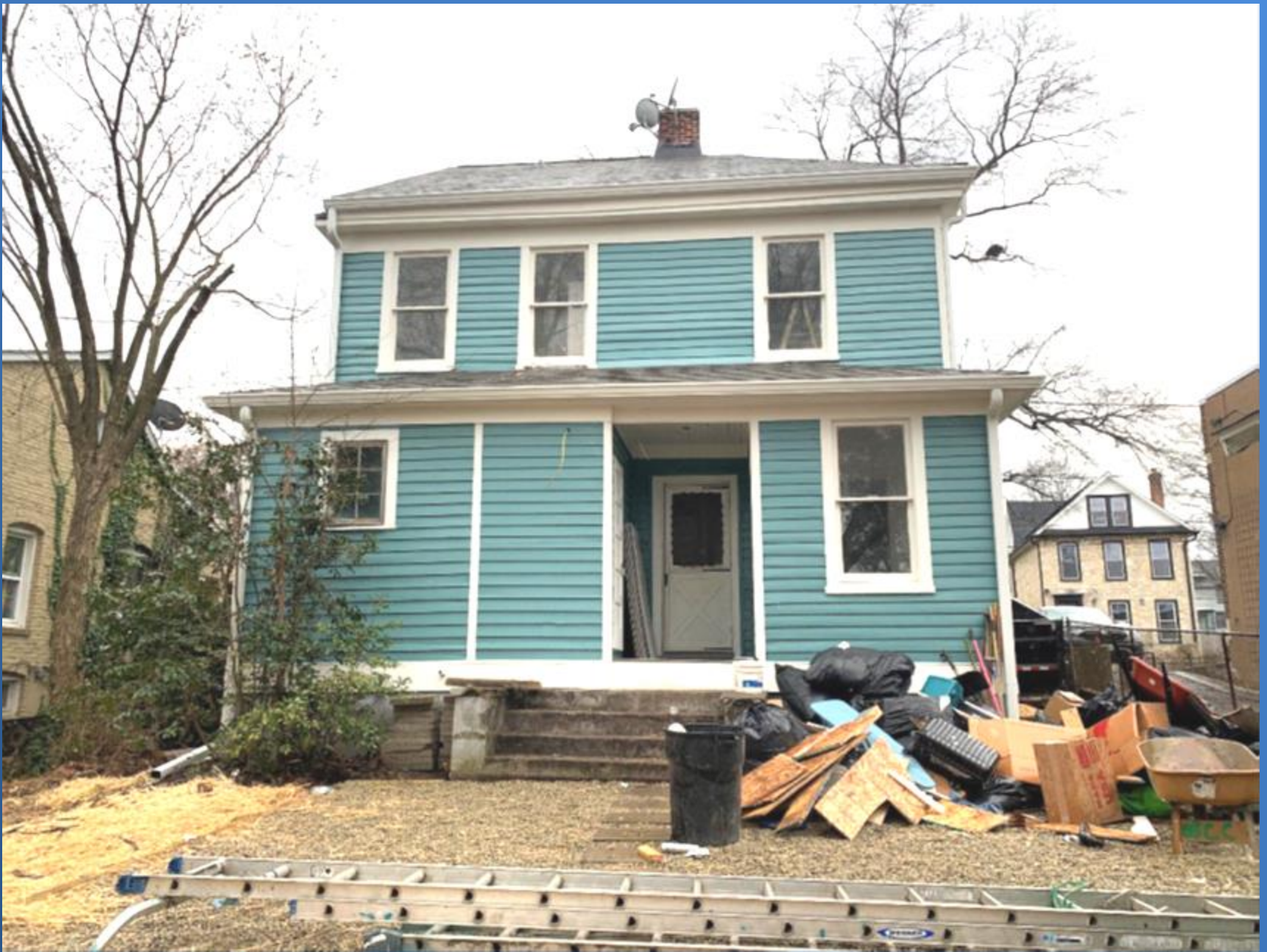
East (rear) elevation, February 2024.
