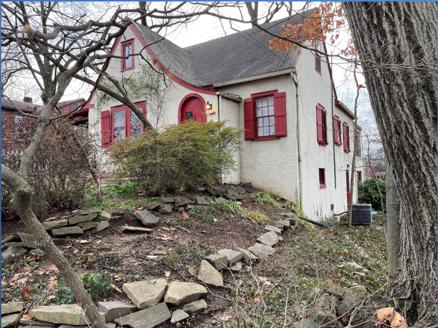
Blair-Smith House, northeast corner, January 2024.
