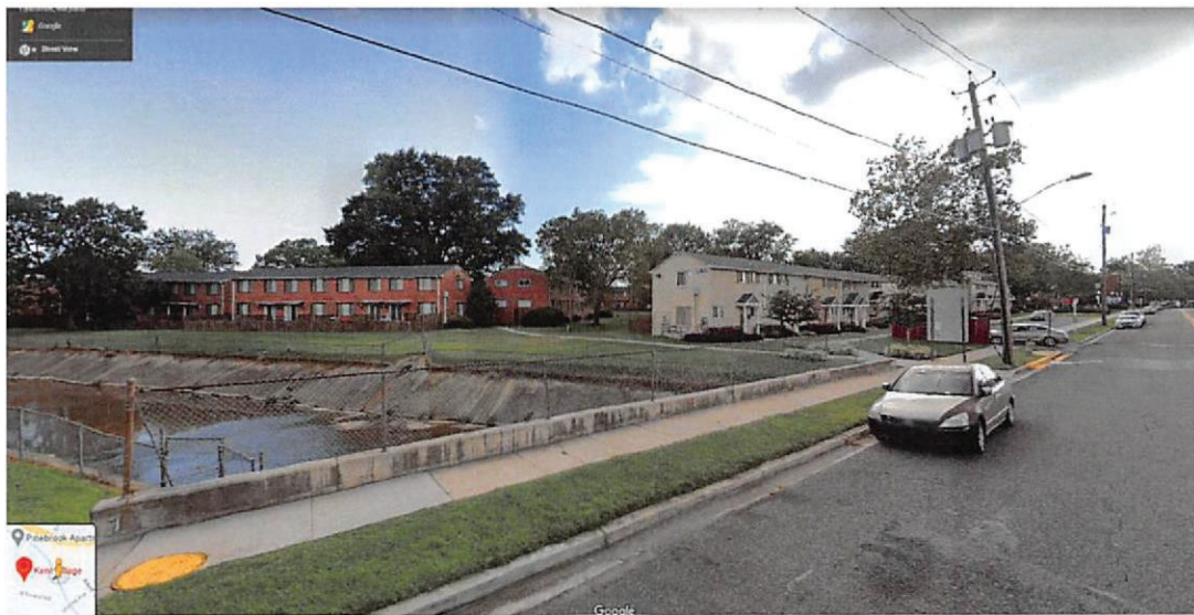
Hawthorne Street looking southwest across the large storm drain facility that bisects Block F. (The playground internal to Block F is not visible).
