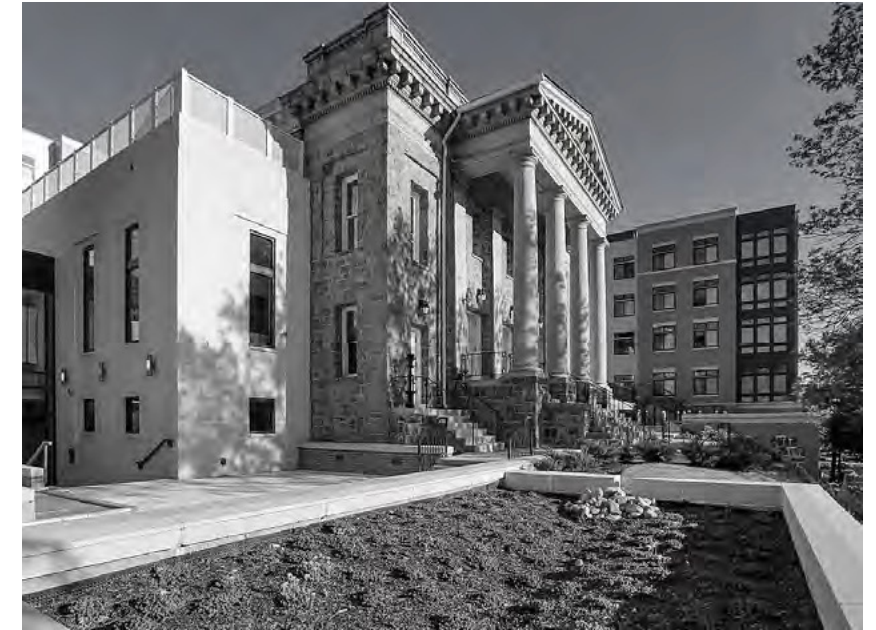
THE BEACON CENTER
