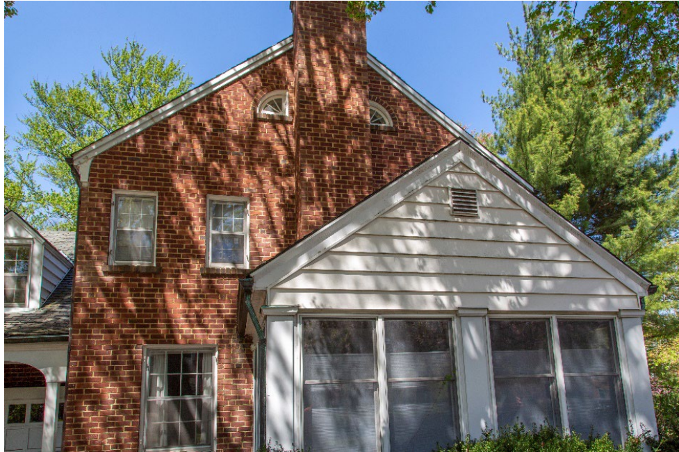
Yates and Mary Boswell House south elevation, April 12, 2023.
