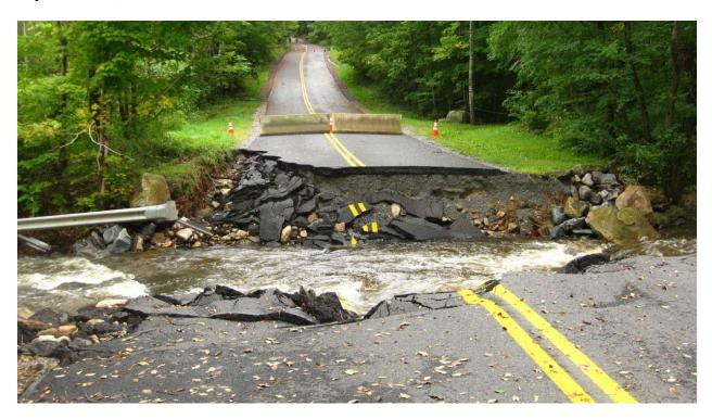
Extreme rain causes culvert washout at Walker Brook in Becket, Massachusetts. (Image credit: Photo courtesy Massachusetts Division of Ecological Restoration.)
