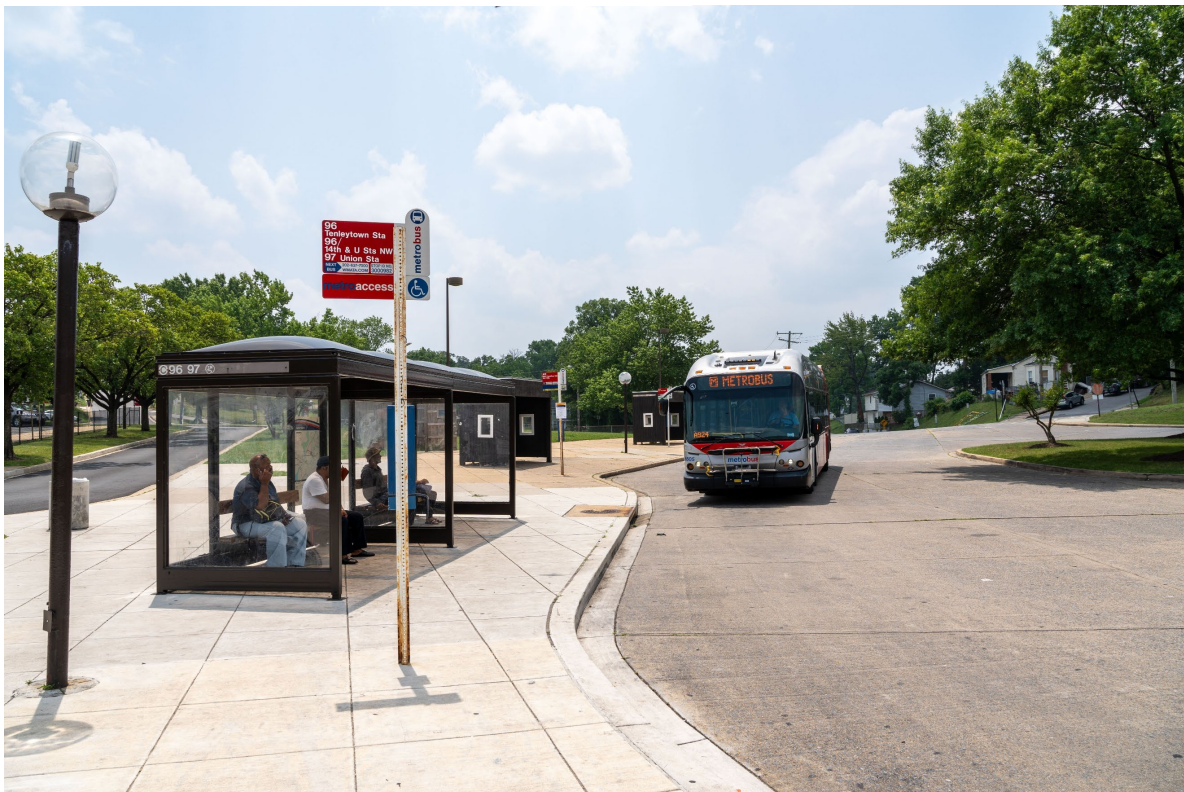
Figure 39. Capitol Heights Metro Station Bus Loop
