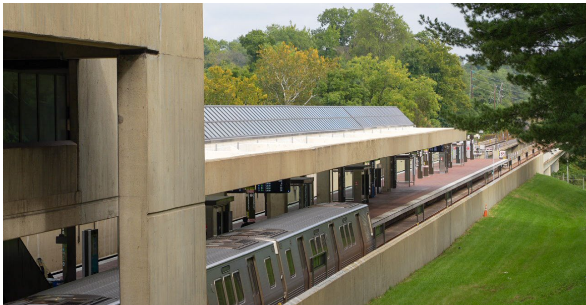
Figure 35. Addison Road-Seat Pleasant Metro Station Platform
