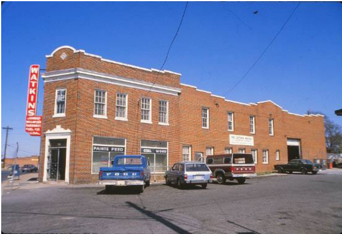
Figure 62. Watkins Hardware Store Building (1986)
