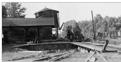
View North, Yard North of Engine House, showing Water Tank and Shop. Photocopy of photograph, 1941 (Courtesy of Chesapeake Beach Railroad Museum; L. W. Rice, photographer) - Chesapeake Beach Railroad Engine House, 21 Yost Place, Seat Pleasant, Prince George's County, MD. Library of Congress (HAER MD-49) .
