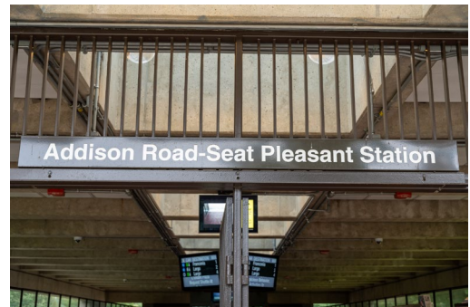
Figure 12. Addison Road-Seat Pleasant Metro Station
