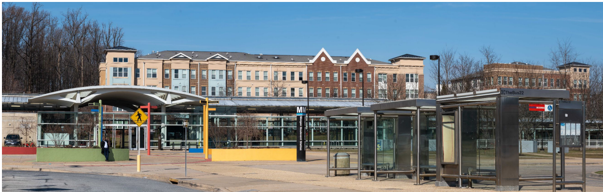
Figure 4. Morgan Boulevard Metro Station
