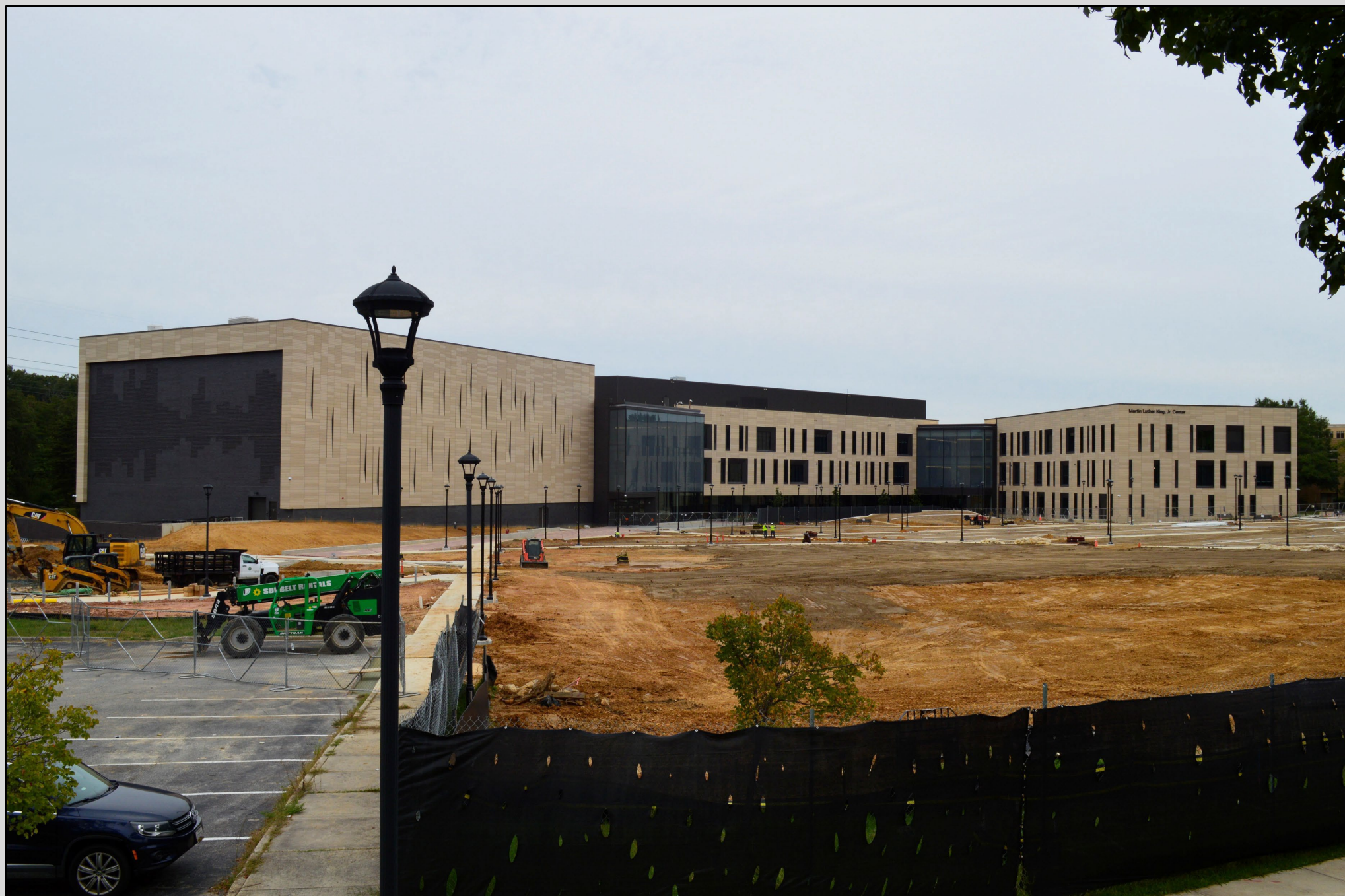
Martin Luther King Jr. Center, adjacent to the MARC Station
