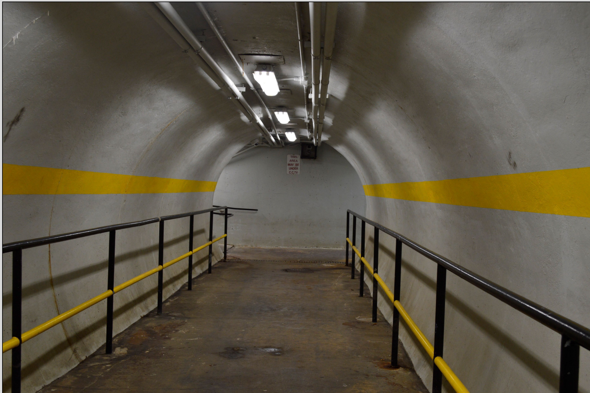
Bowie State MARC Station Tunnel
