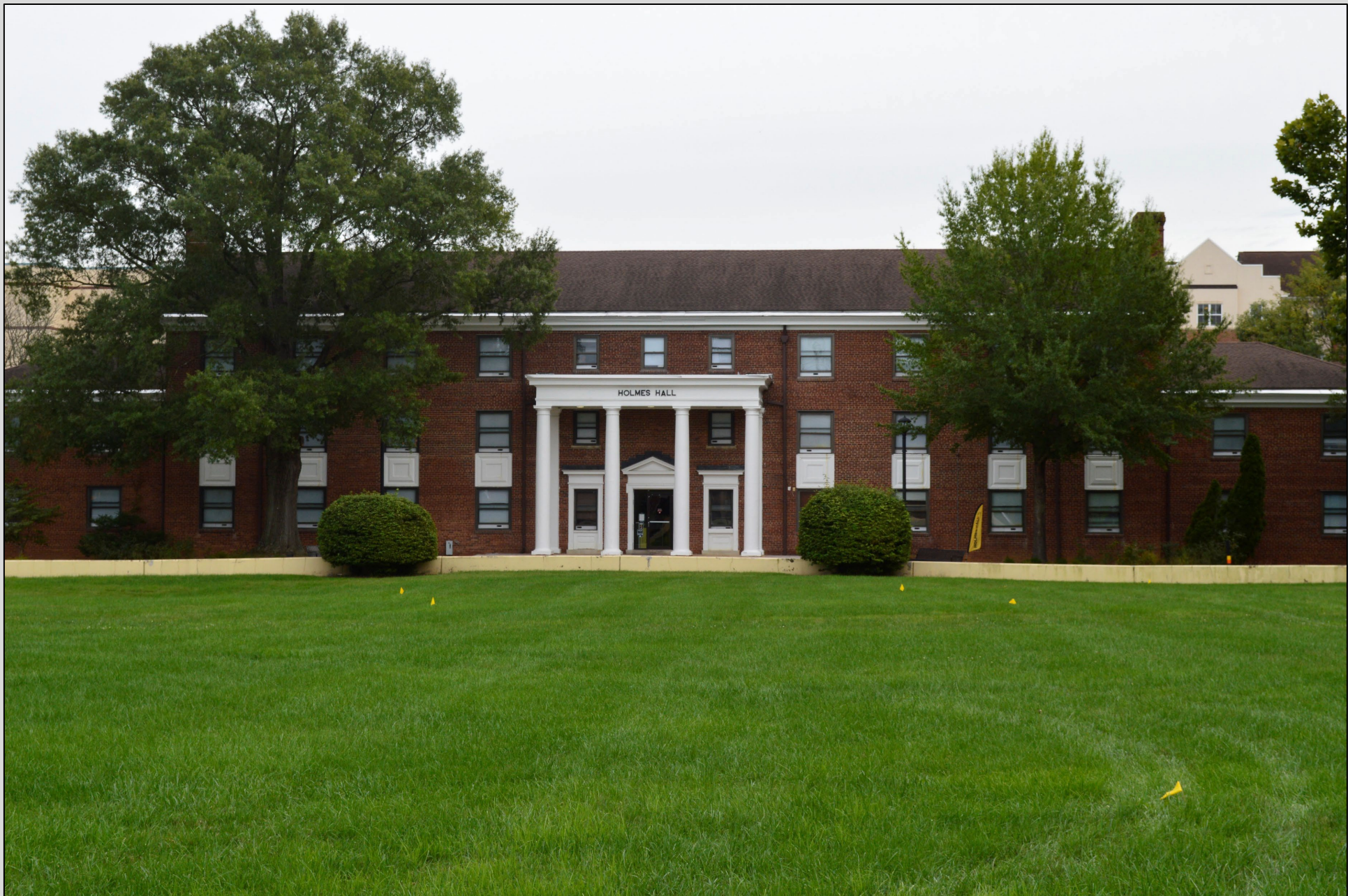
Dwight Oliver Holmes Hall, an all-male traditional three-story residence hall with double rooms, community bathrooms and showers
