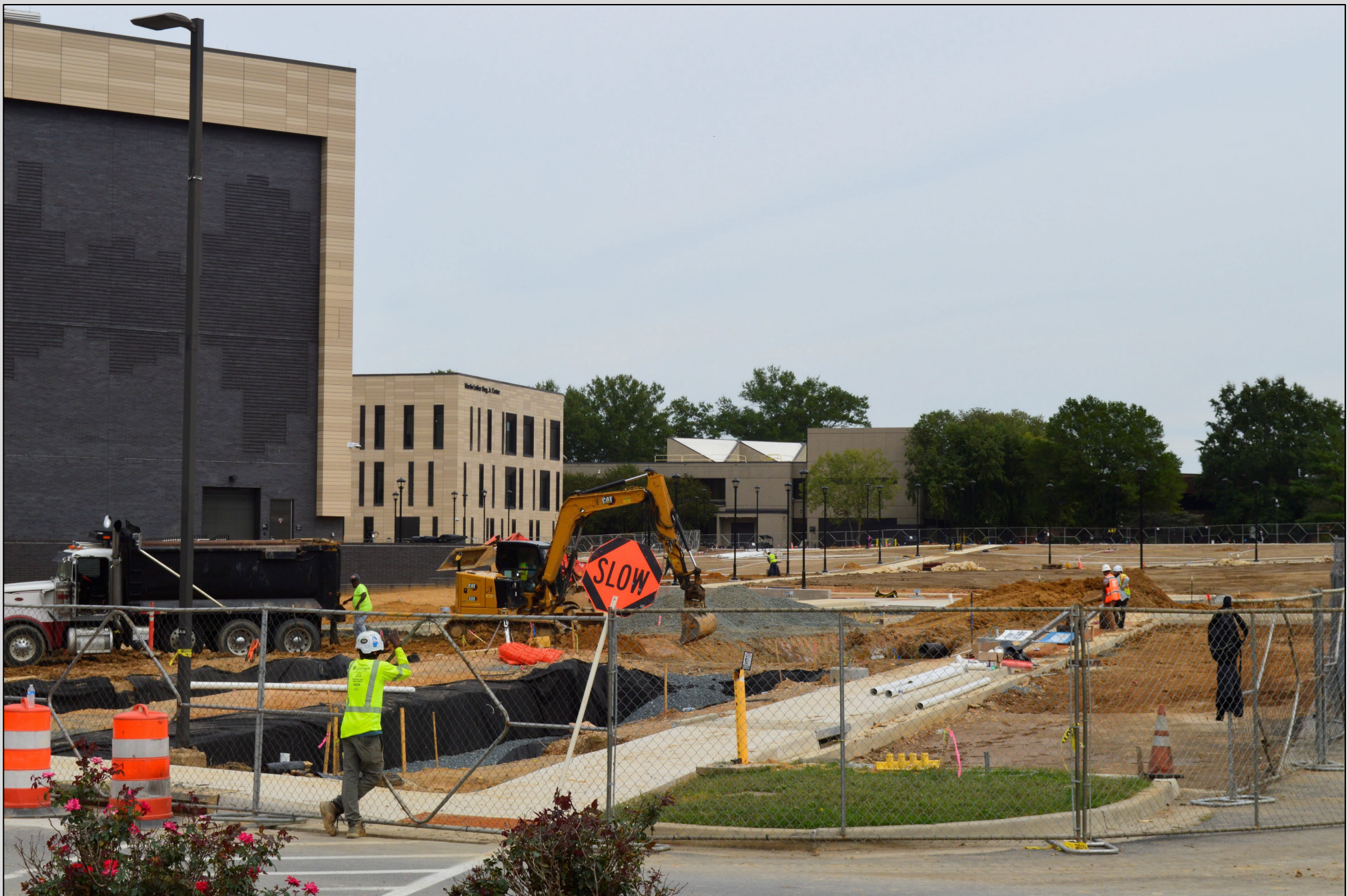
Construction of BSU's new library is underway, adjacent to the MARC Station.
