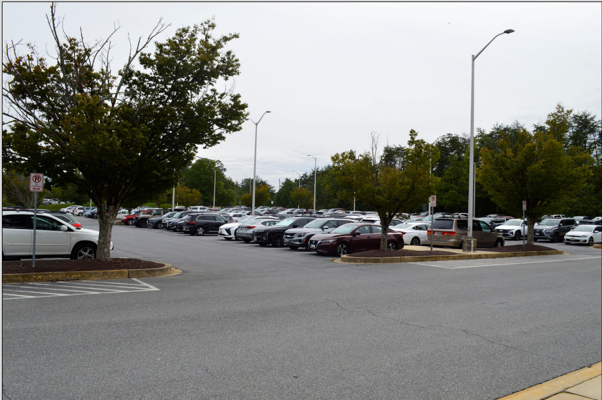
East parking lot (BSU side) of Bowie State MARC Station
