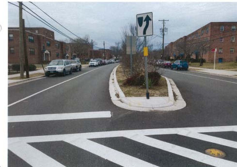
Merrimac Drive - After
