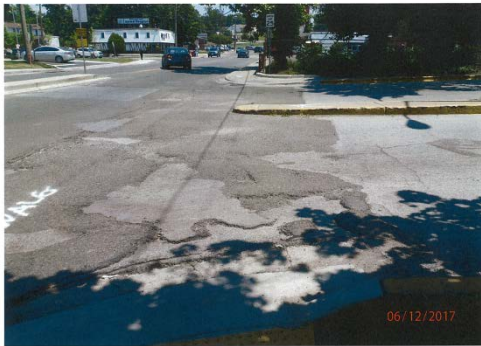
Kenilworth Avenue @ Riverdale Road - Before
