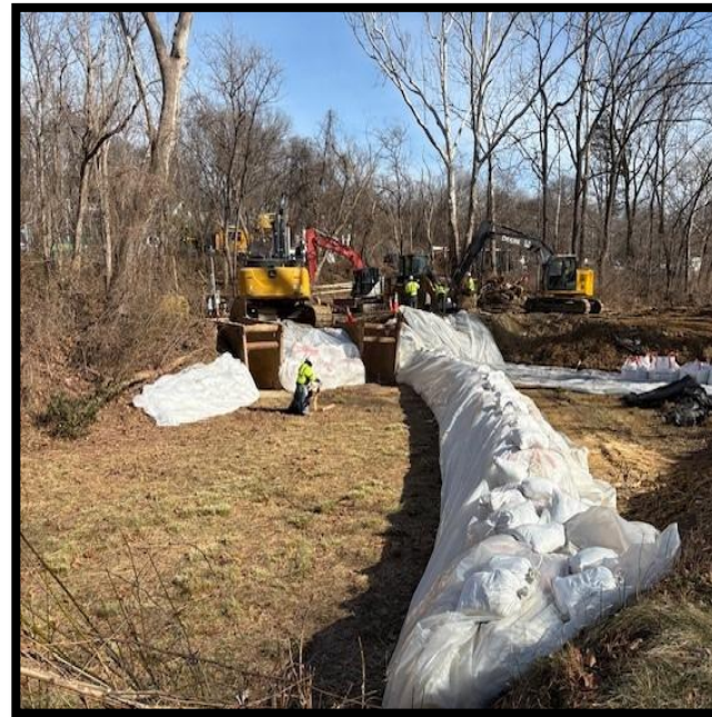
Coffer Dam in Canal
