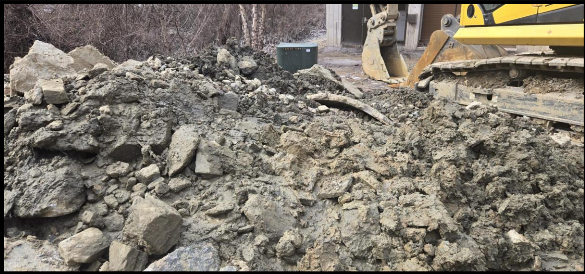
Rocks and boulders removed from the Interceptor and above the pipe
