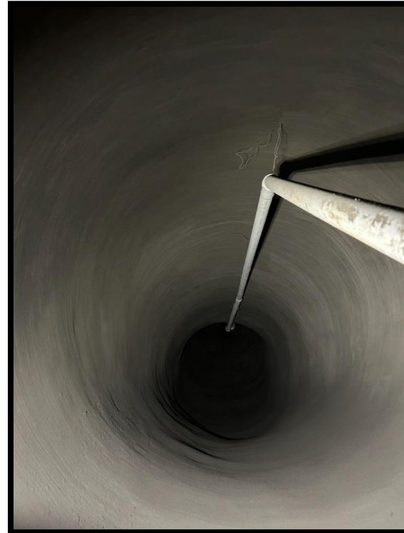
Pipe Strengthened with Geopolymer
