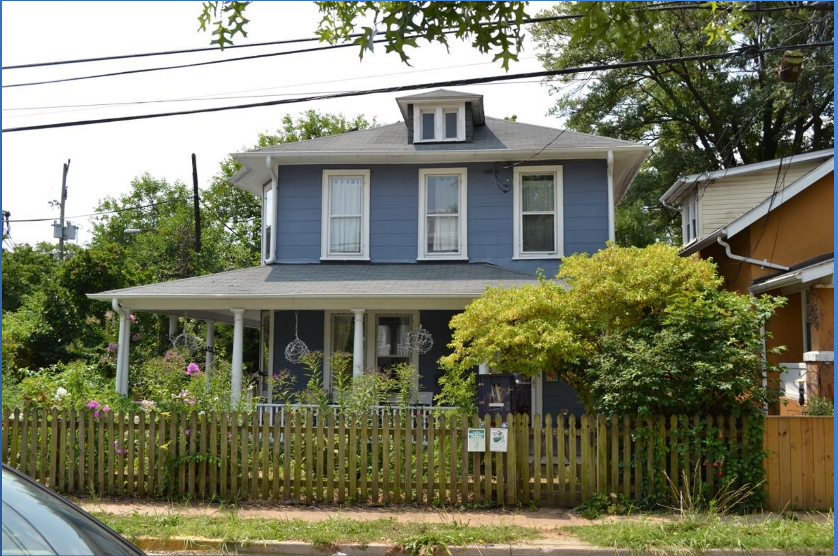
Edward & Maggie Smith House, North Elevation, July 2021
