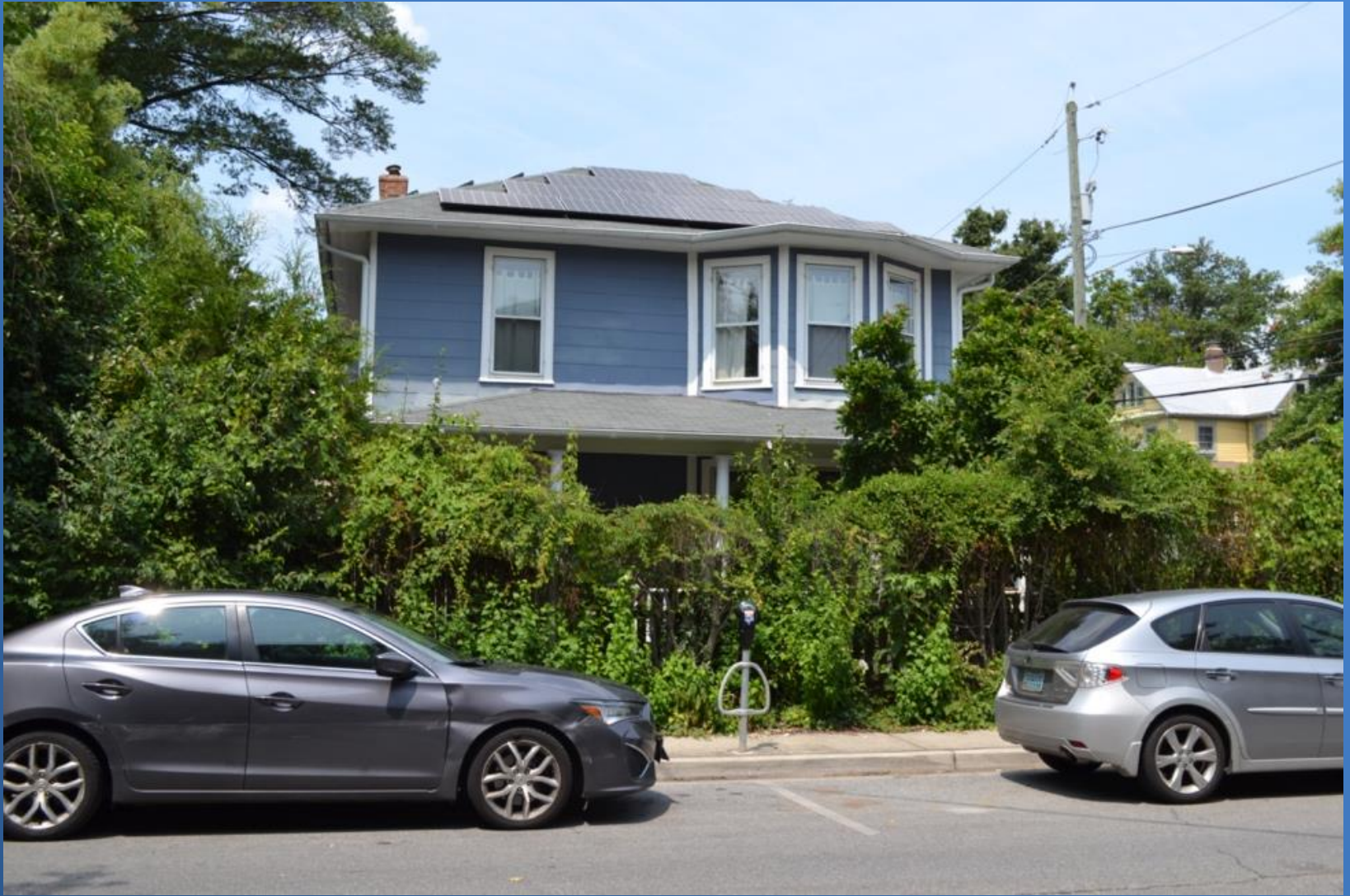
Edward & Maggie Smith House, East Elevation, July 2021
