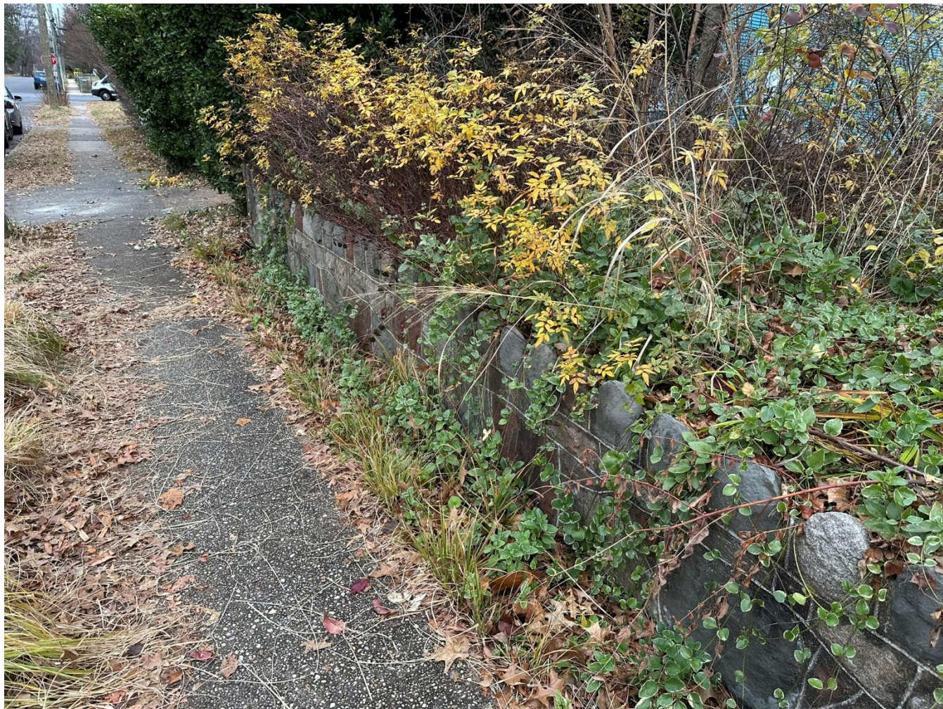
Weinstein House/Harry's Market, Stone retaining wall at east property line, November 25, 2025
