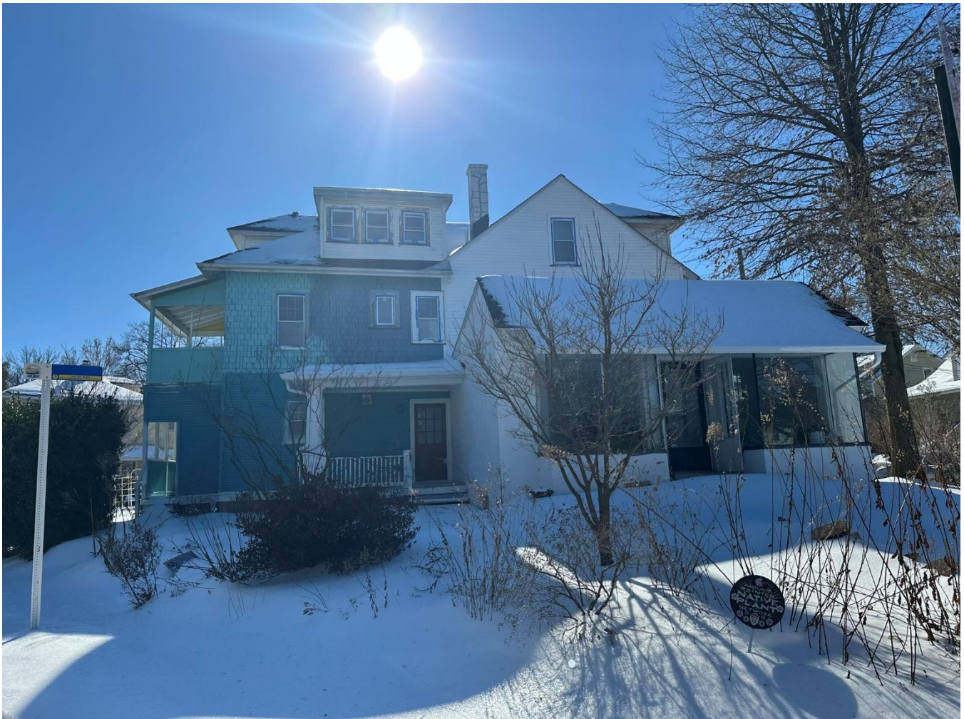
Weinstein House/Harry's Market, North Elevation, February 2, 2026.
