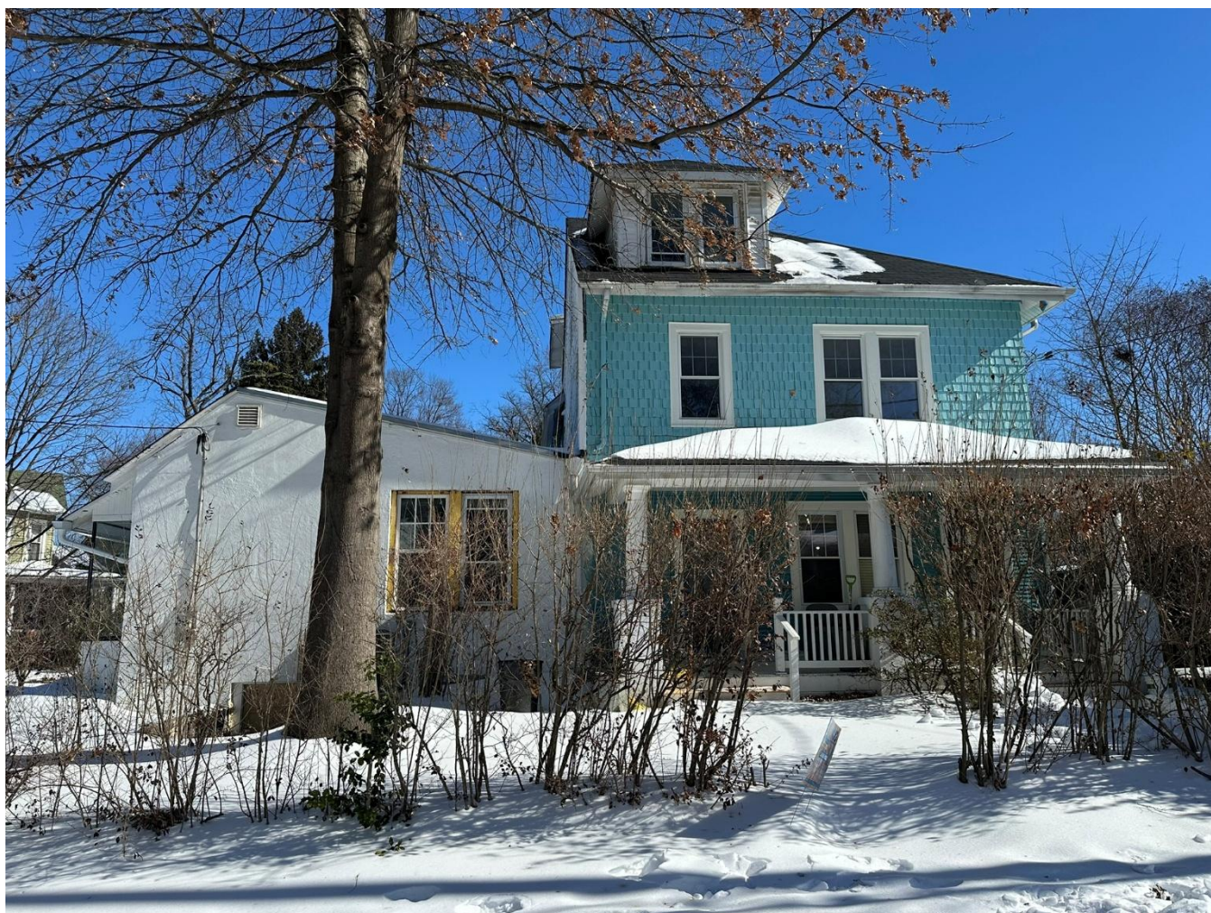
Weinstein House/Harry's Market, West Elevation, February 2, 2026.
