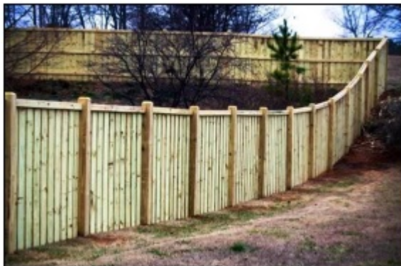
Figure 27-6606(a): Fence with Finished Side Out
