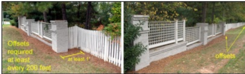
Figure 27-6605(c): Fence and Wall Offsets
