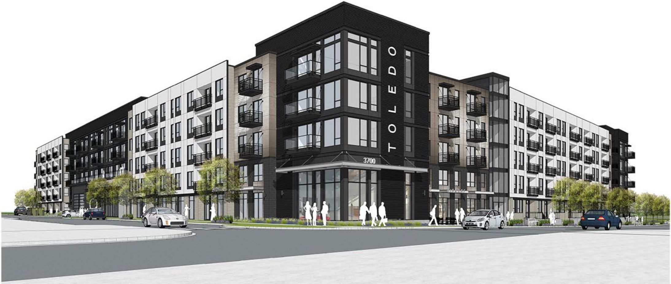
V1 - CORNER OF TOLEDO RD. & NEW STREET
