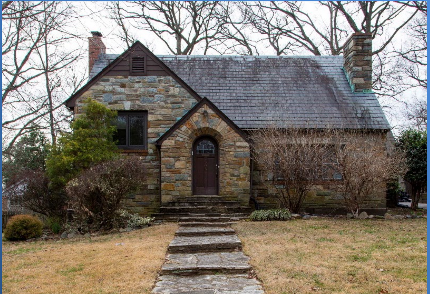
North (front) elevation, February 2020.
