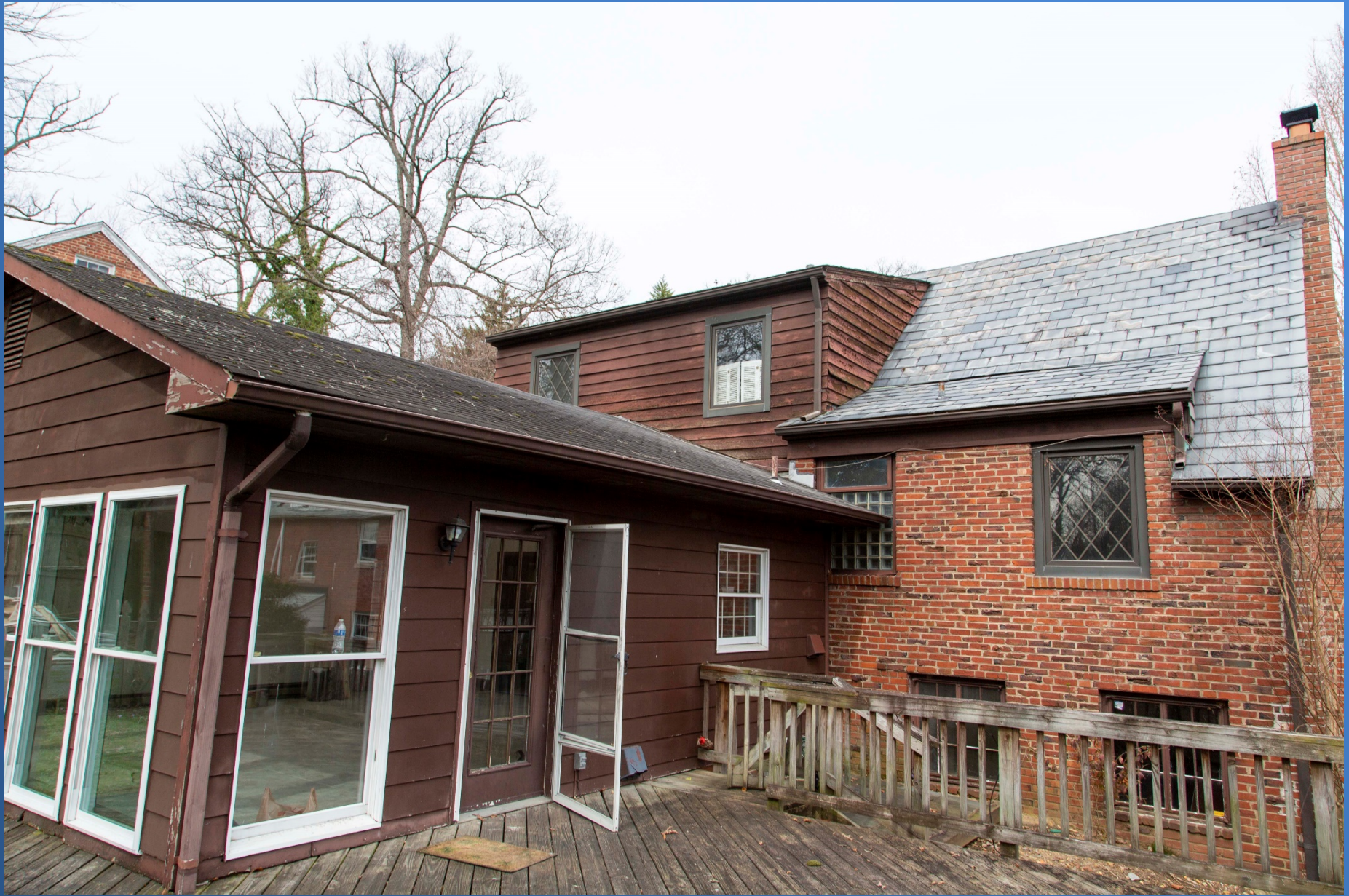
Southeast corner, February 2020.
