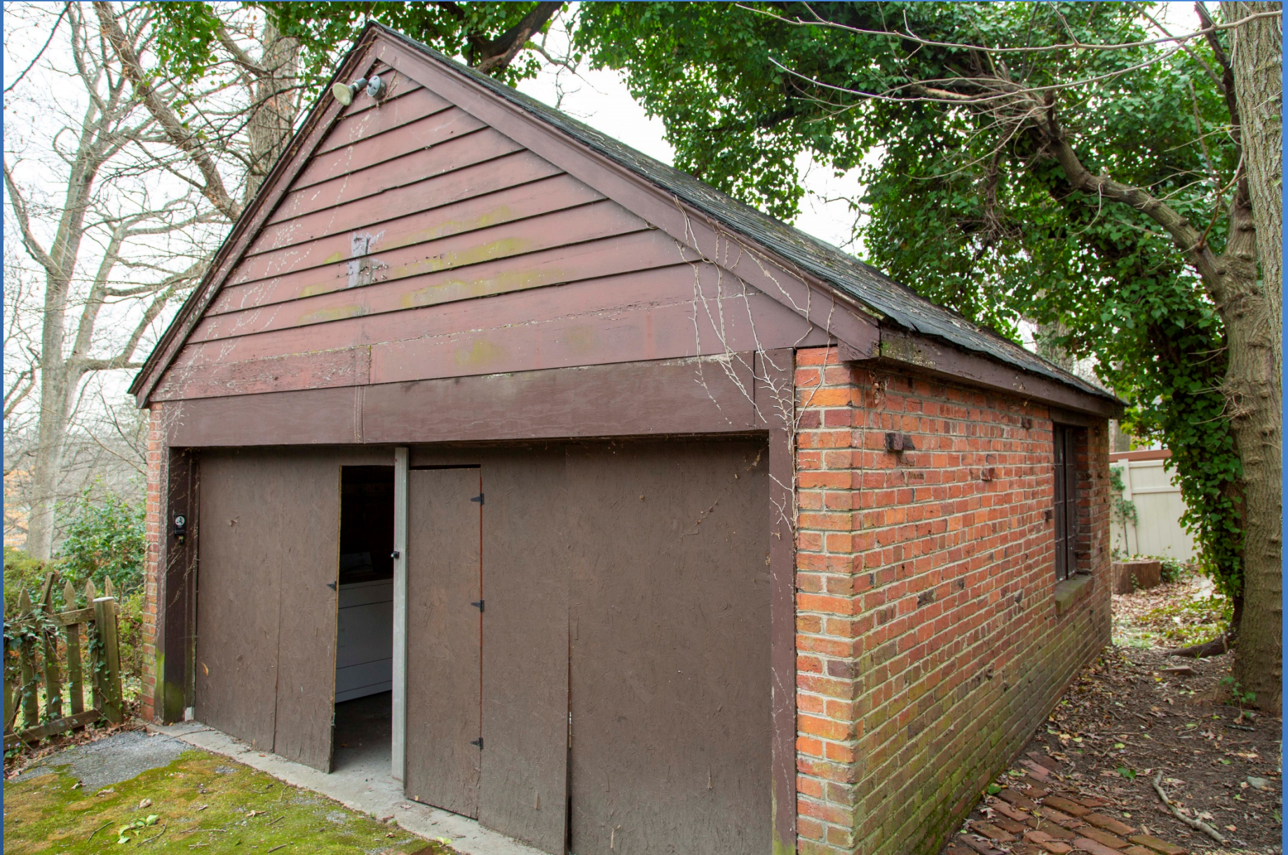
Garage northwest corner, February 2020.
