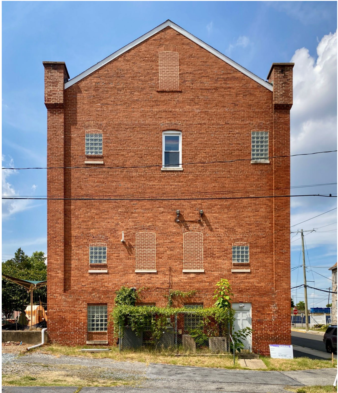
Mount Harmon Lodge Masonic Temple, south elevation, July 8, 2024.
