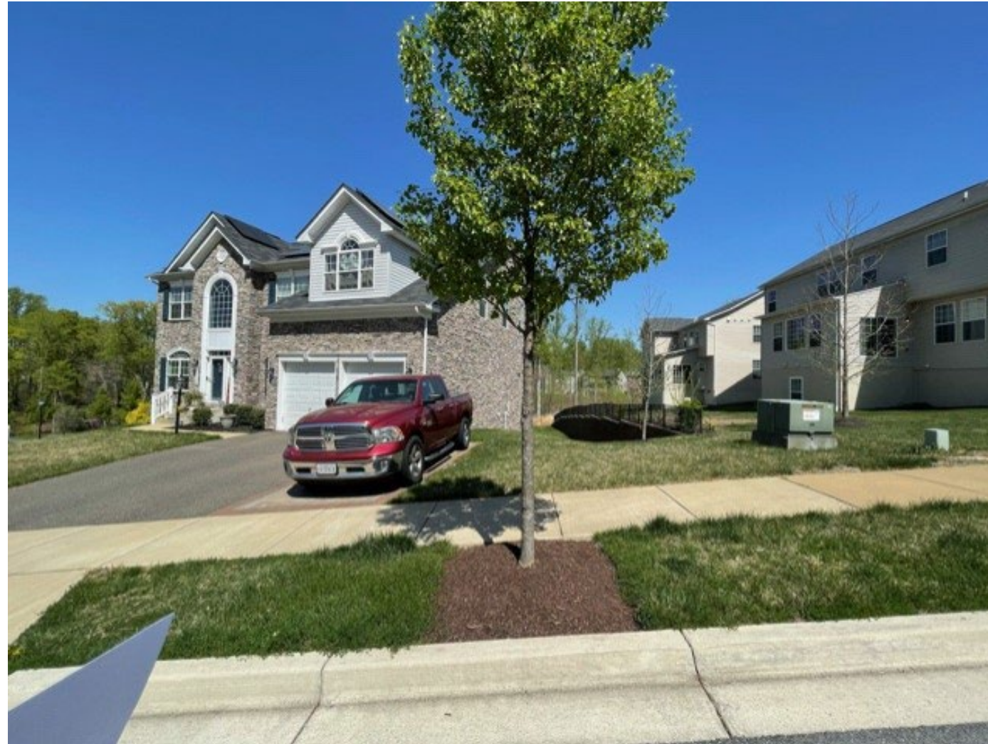
Front View of Existing Property
