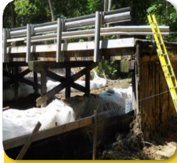
Bridge Repair, Reconstruction And Construction
