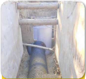
Storm Drain Improvement and Culvert Repair
