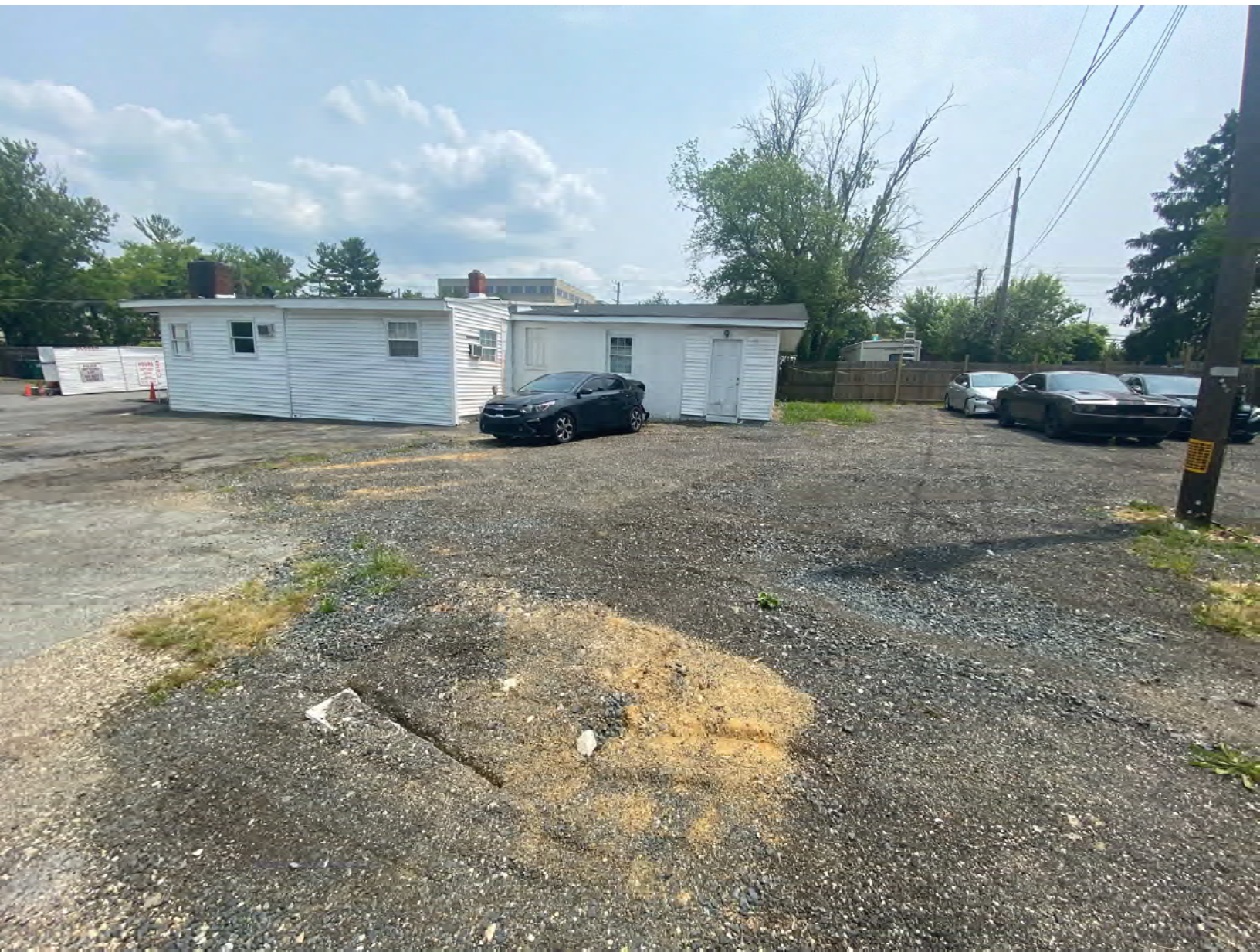
Rear of main building
