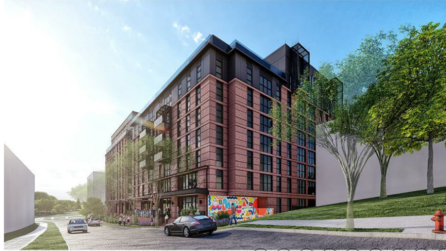
VIEW LOOKING NORTHWEST FROM KNOX ROAD
