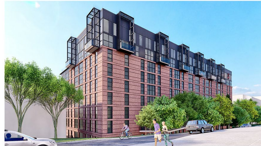
VIEW LOOKING SOUTHWEST FROM LEHIGH ROAD
