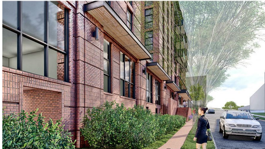
VIEW LOOKING EAST ALONG KNOX ROAD
