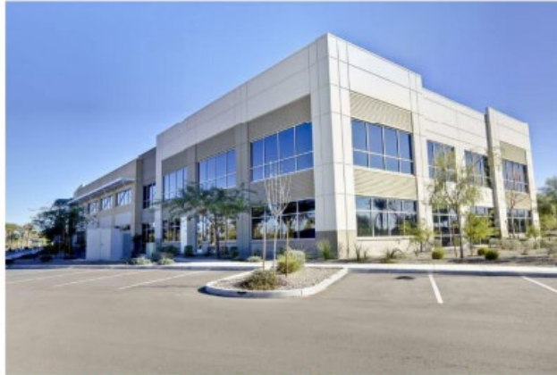
EXAMPLE OF MASSING AND MATERIALS- LARGE AMOUNTS OF GLAZING, FORMLINER AT WINDOWS
