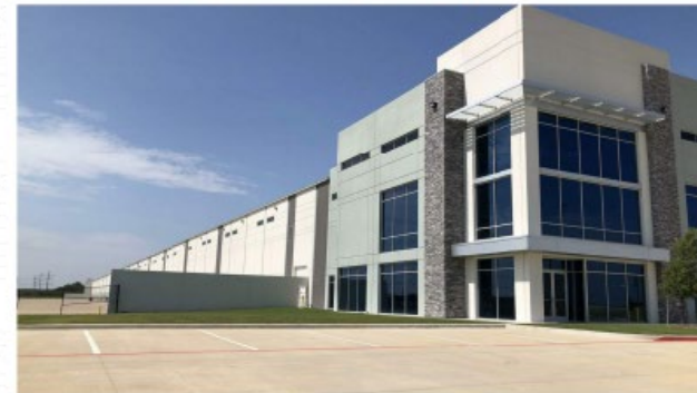
EXAMPLE OF MASSING AND MATERIALS- ALUMINUM SUNSHADES
