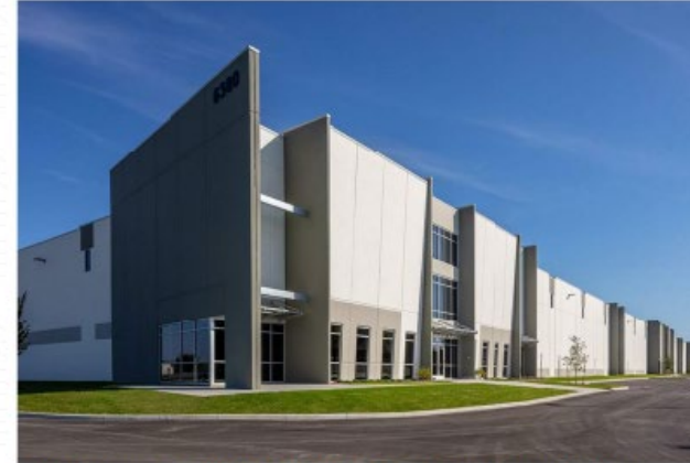
EXAMPLE OF MASSING AND MATERIALS- VERTICAL FINIS, PAINTED CONCRETE TILT UP PANELS
