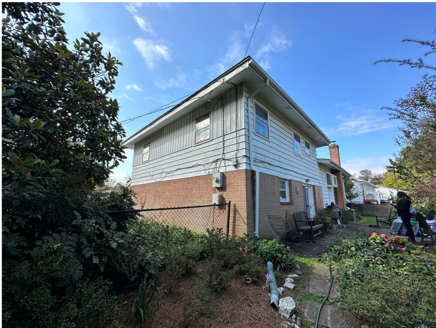
Figure 7: Northeast corner, 5110 Pierce Avenue.
