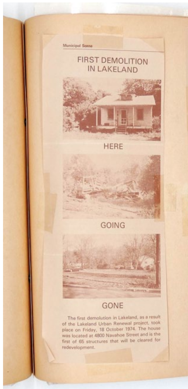
Figure 21: The Lakeland Urban Renewal project began demolitions in 1974. Excerpt, Edwards Scrapbook (1969-1979), Lakeland Digital Archive.
