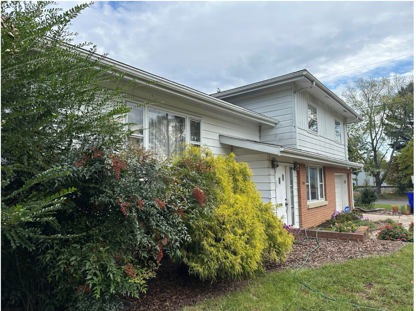
Figure 3: Southwest corner, 5110 Pierce Avenue.
