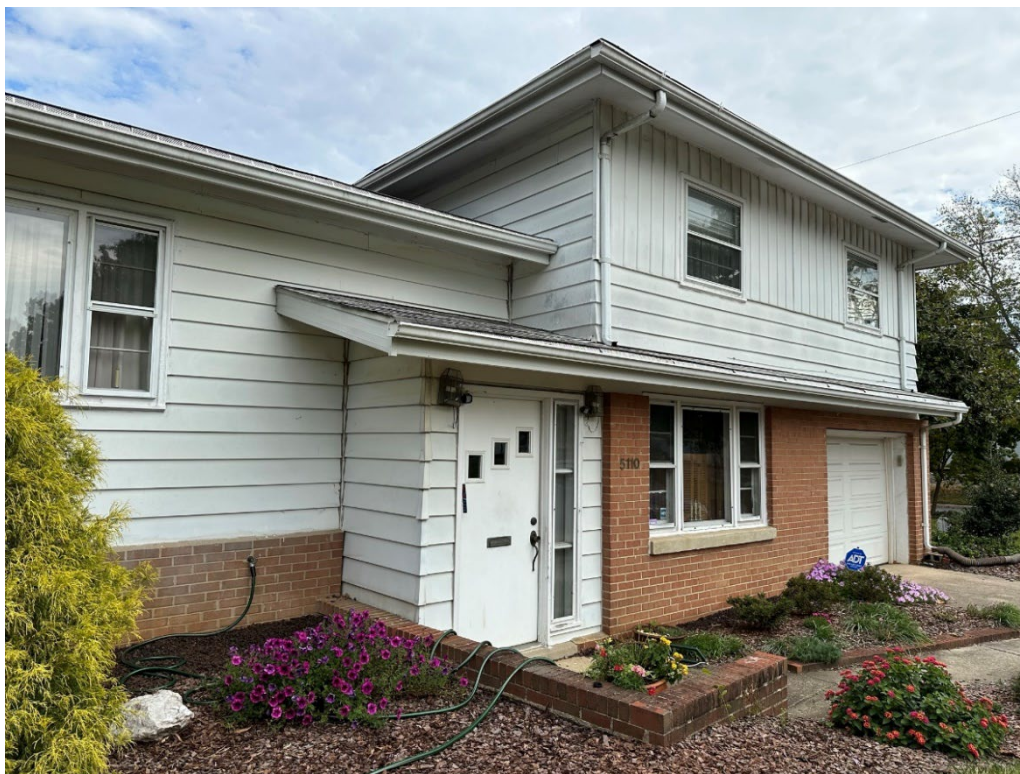
Figure 2: Elwood and Wilmer Gross House, south elevation looking northeast, October 2023.
