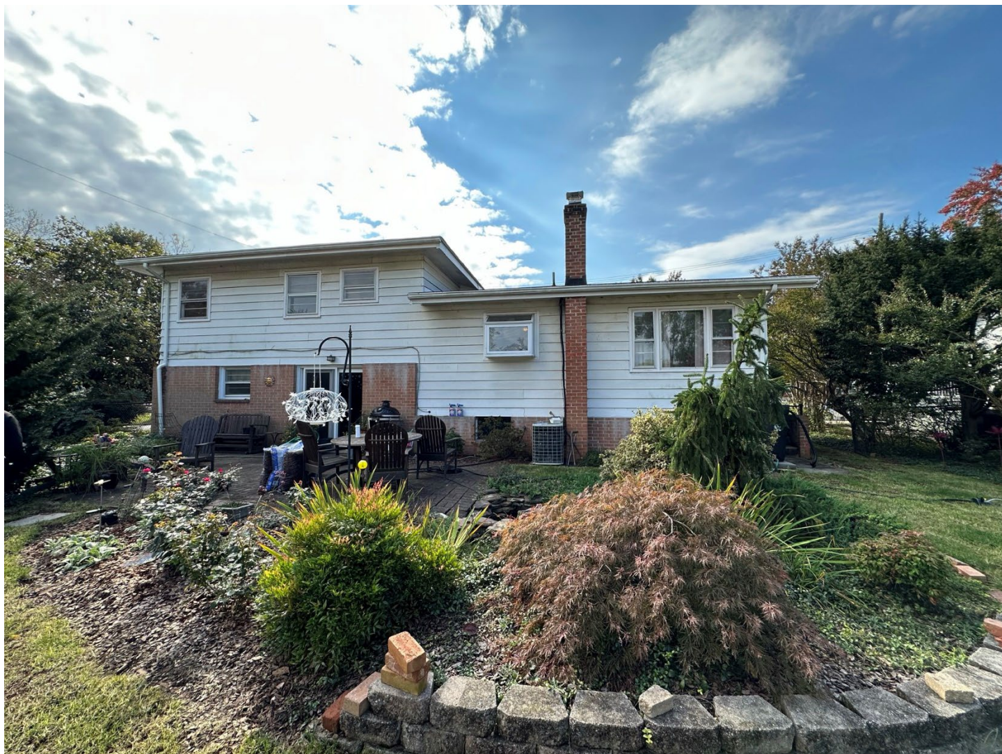
Figure 5: North elevation (rear), 5110 Pierce Avenue.
