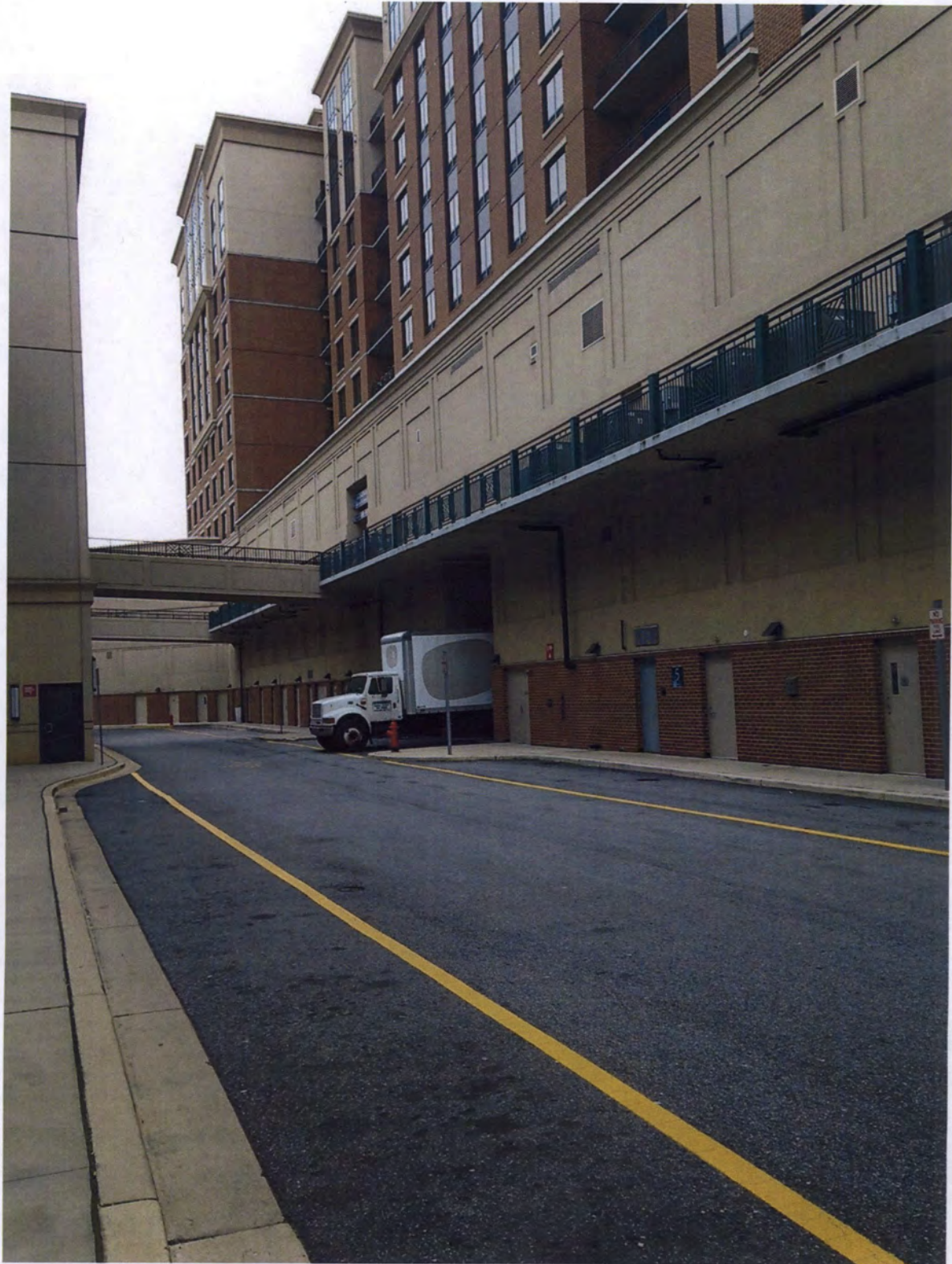
This internal road at the Annapolis Towne Centre at Parole accommodates sidewalks along both sides by placing the switchyard at the second level above the sidewalk (see above on the right side of the road).
