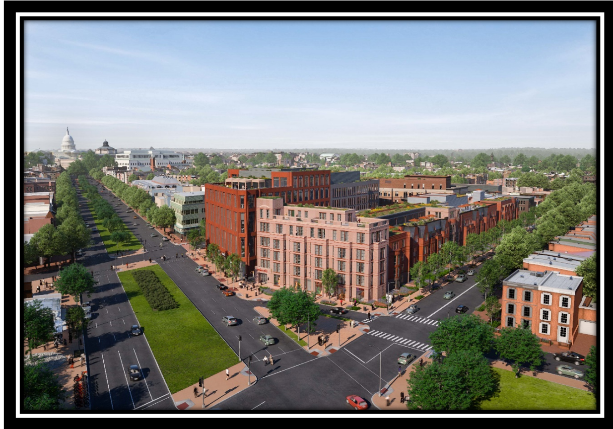
Hine Middle School Redevelopment, Eastern Market Metro Station
