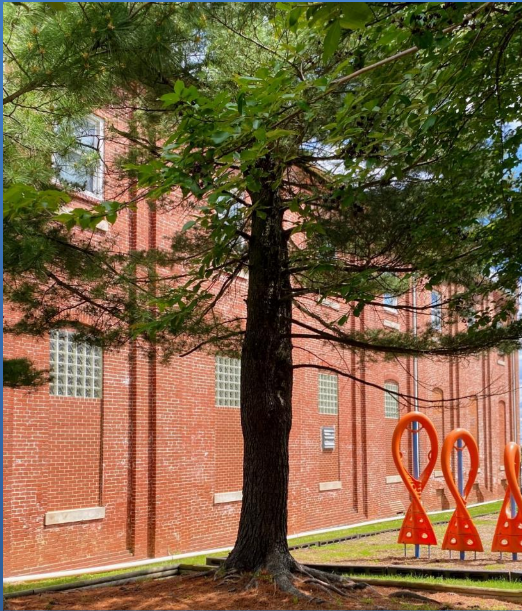
Partial view of west elevation, May 2024.
