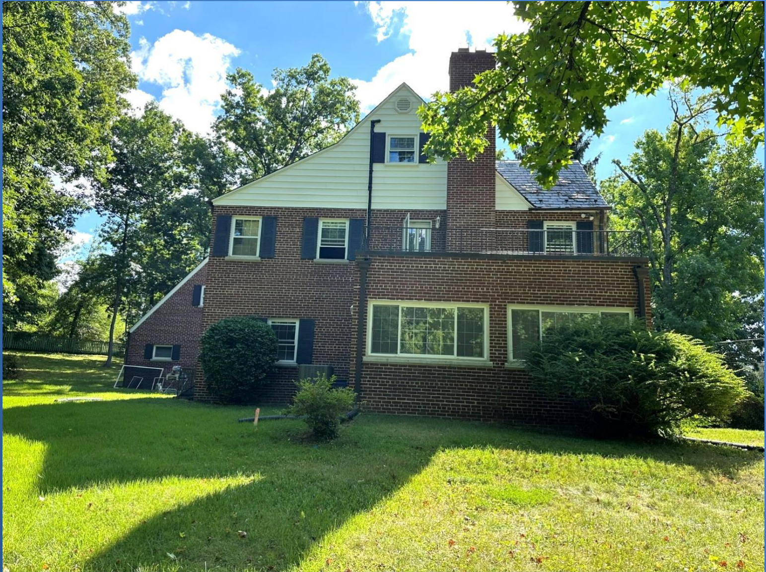
West Elevation June 24, 2024
