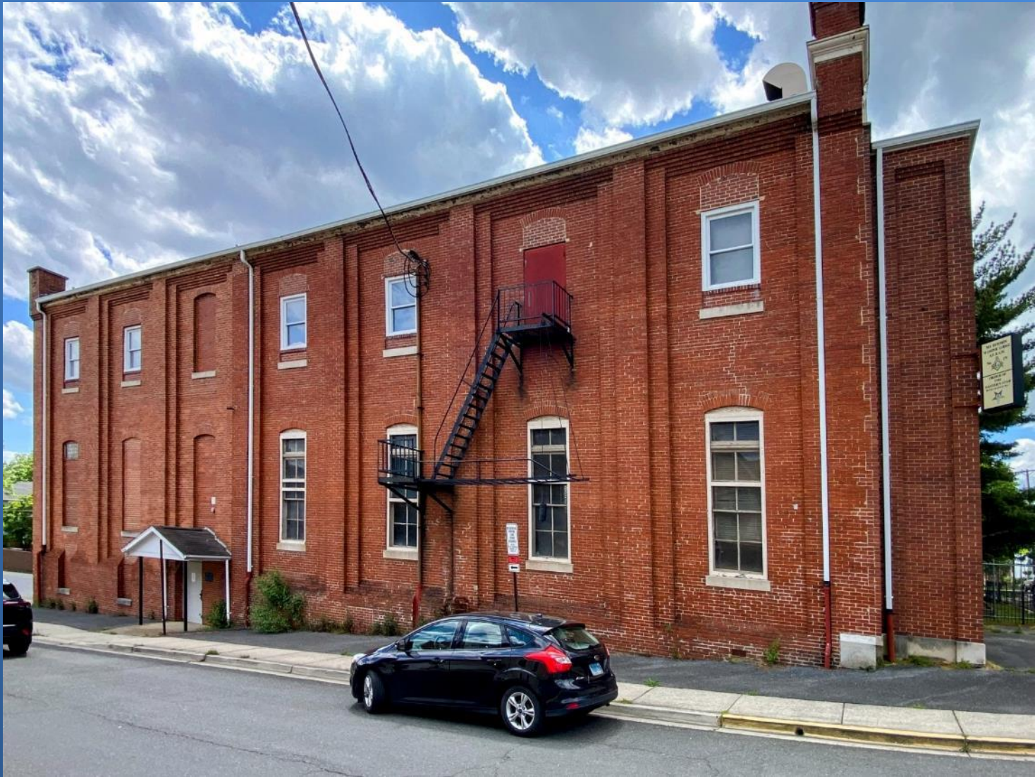
East elevation, May 2024.
