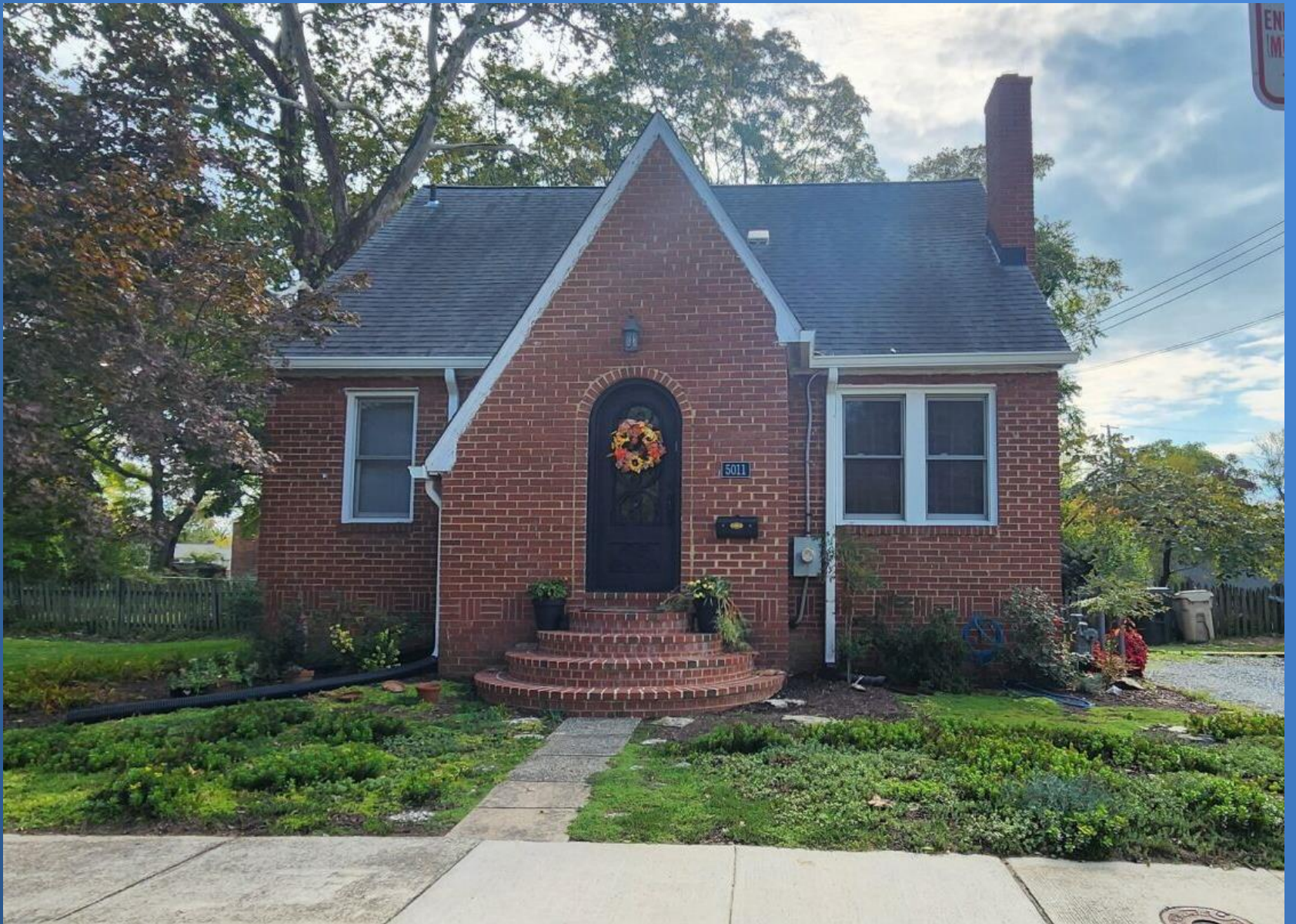
North (Front) elevation, November 2023
