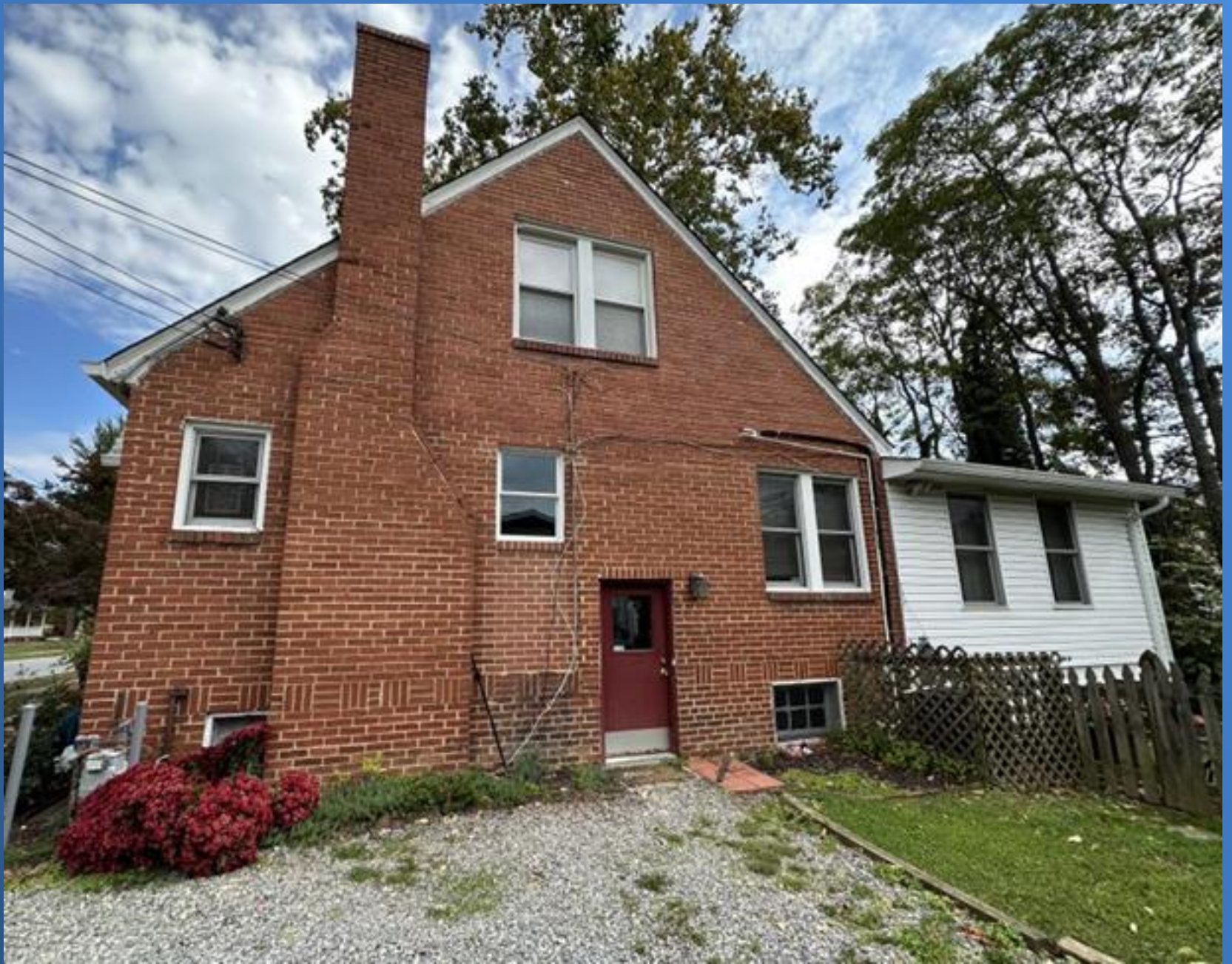
West elevation, November 2023
