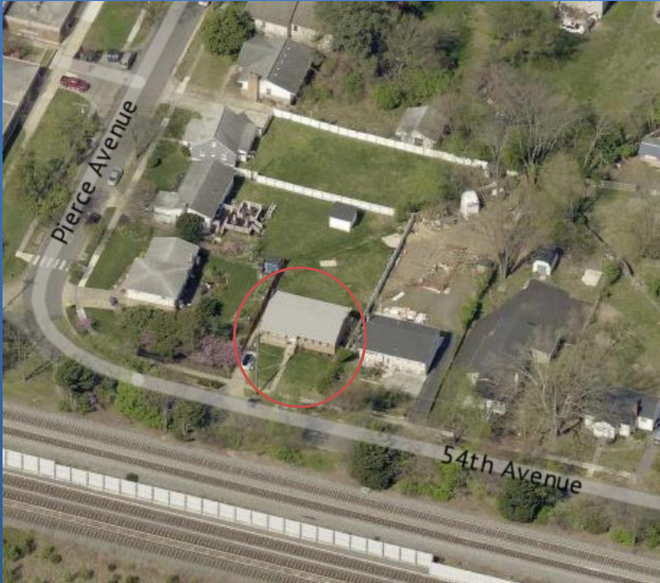
Oblique aerial view from east, December 2021. Pictometry via PGAtlas.com
