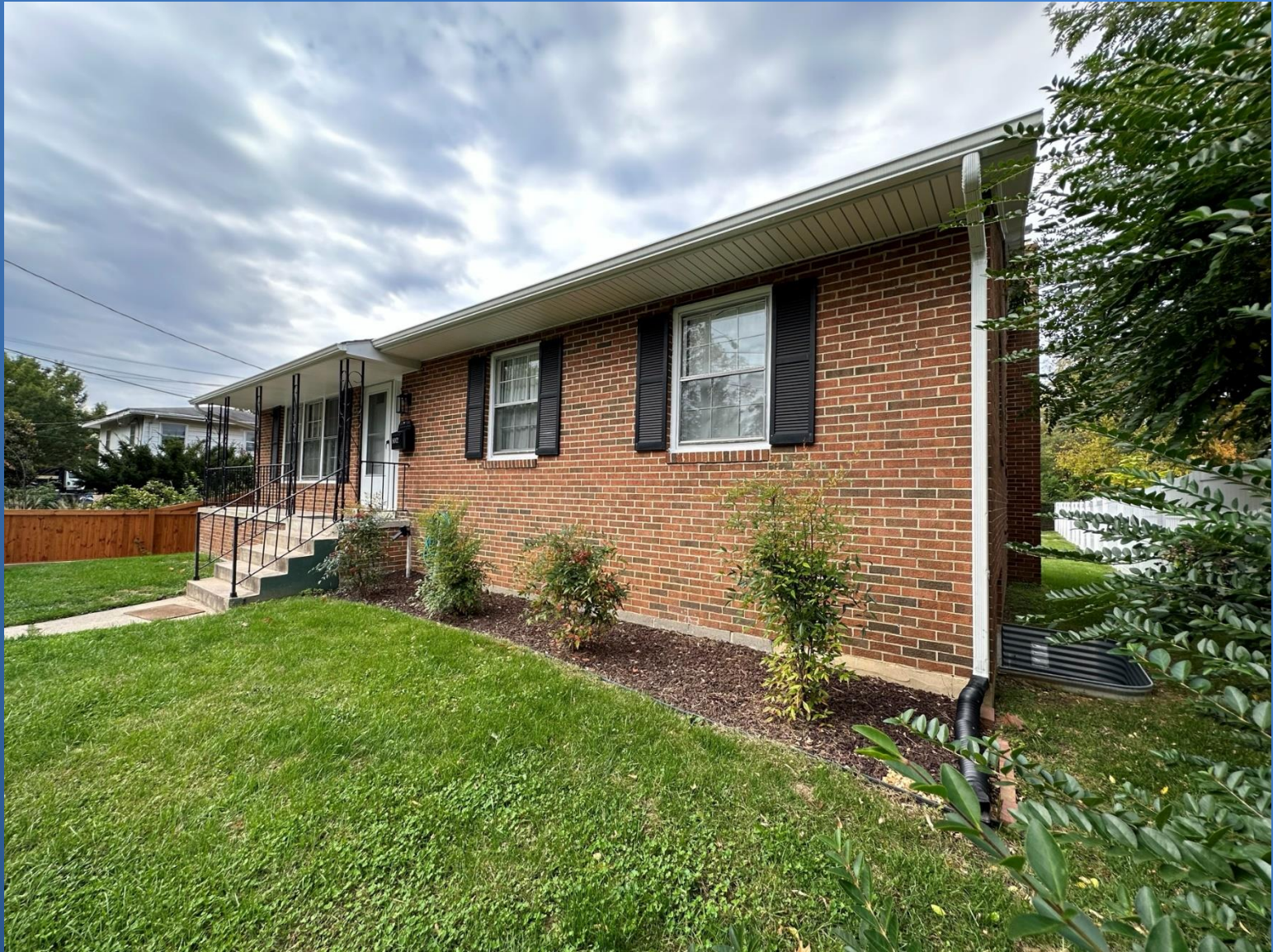
Northeast corner, October 2023.
