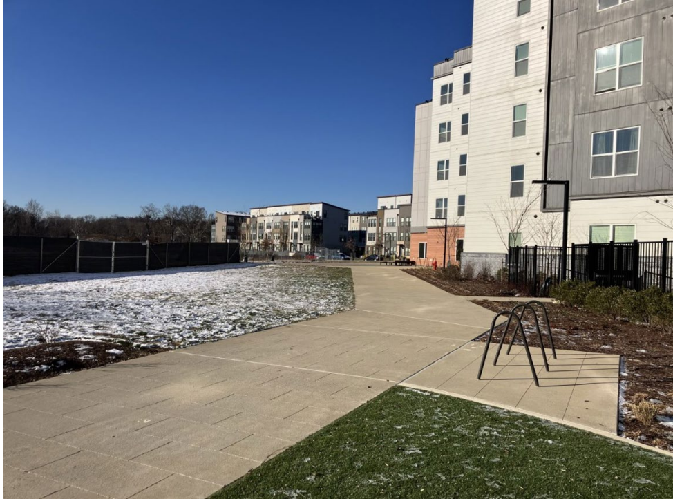
EXISTING PEDESTRIAN PROMENADE
