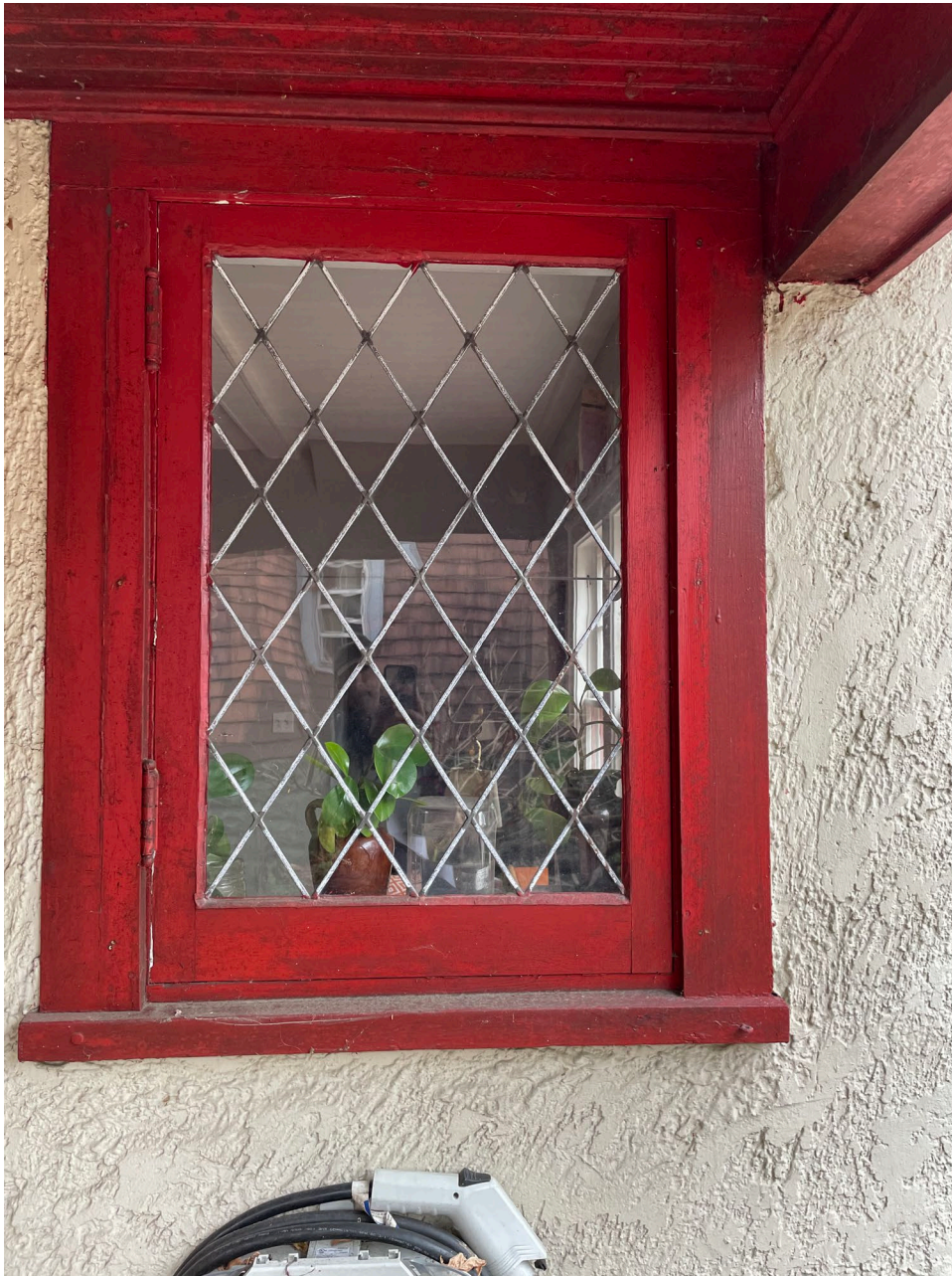
Figure 6: Casement window in south elevation (side porch) of 5416 39 th Avenue
