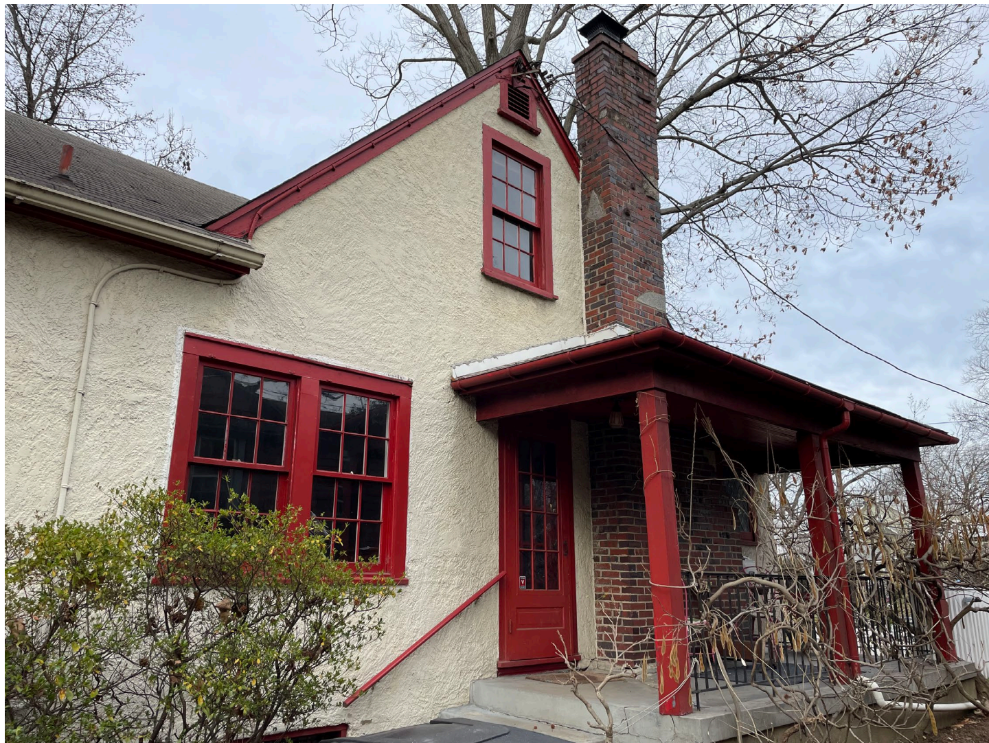
Figure 2: The south elevation of 5416 39 th Avenue.
