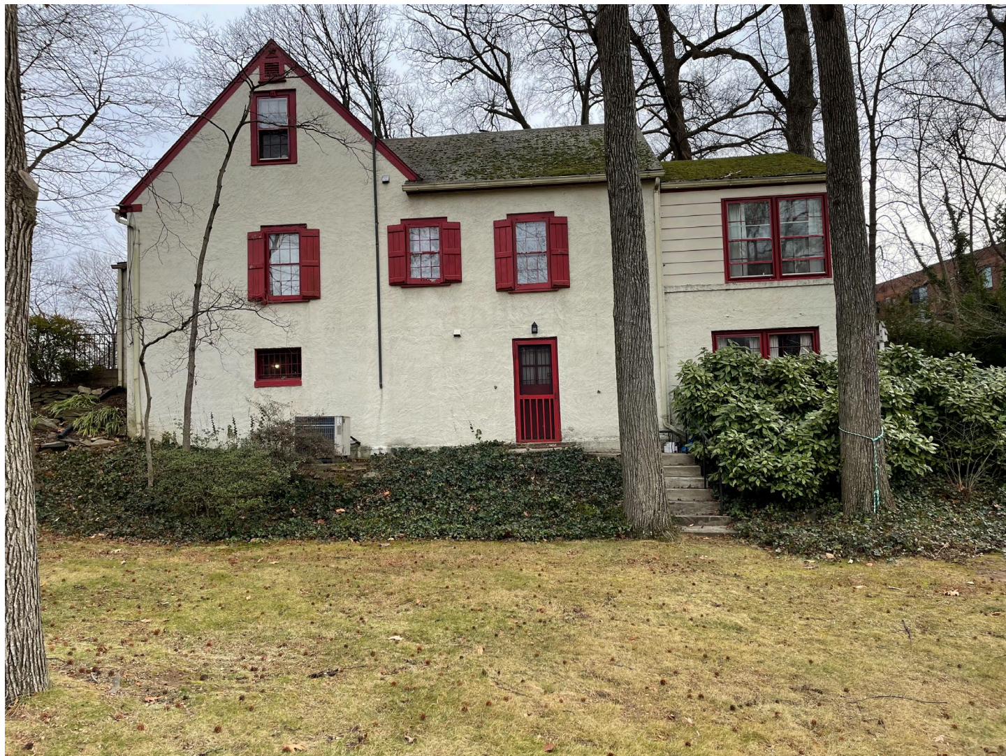
Figure 4: The north elevation of 5416 39 th Avenue.
