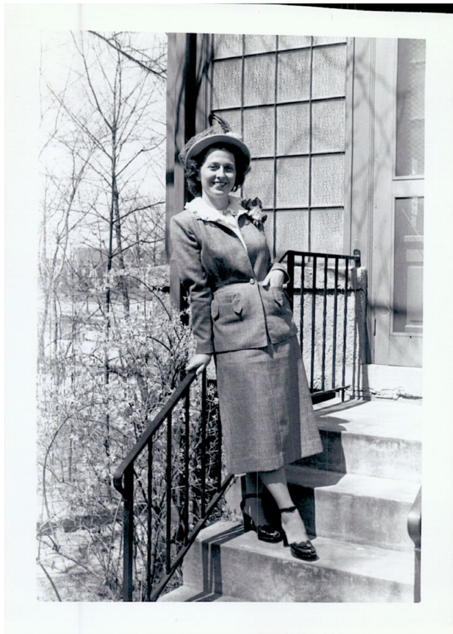
Figure 13. Geraldine Smith on stairs of the rear sunroom addition.
