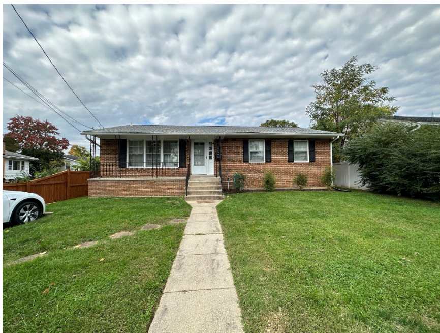
Figure 1: East elevation (façade), 8002 54 th Avenue.
