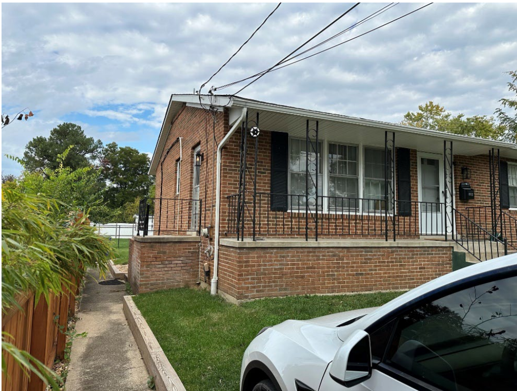
Figure 2: Southeast corner, 8002 54 th Avenue, October 2023.
