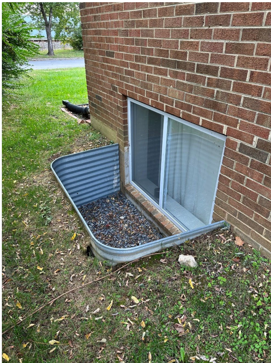
Figure 9: Basement egress window, northwest corner, 8002 54 th Avenue.
