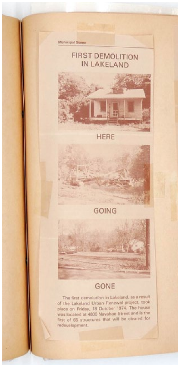
Figure 24: The Lakeland Urban Renewal project began demolitions in 1974. Excerpt, Edwards Scrapbook (1969-1979), Lakeland Digital Archive.
