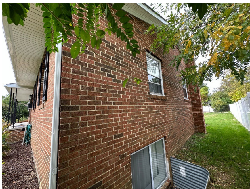
Figure 8: Northeast corner, 8002 54 th Avenue.
