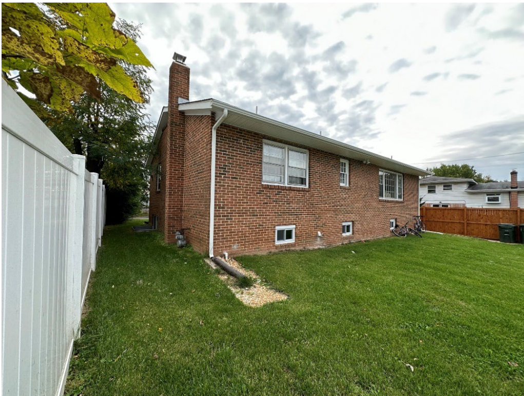
Figure 4: Northwest corner, 8002 54 th Avenue, October 2023.
