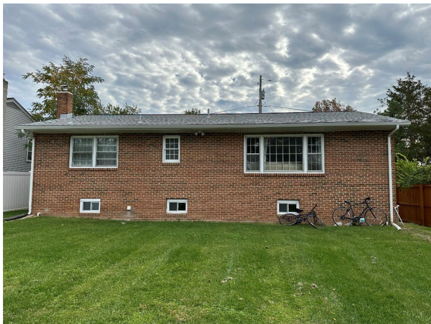
Figure 5: West (rear) elevation, 8002 54 th Avenue.
