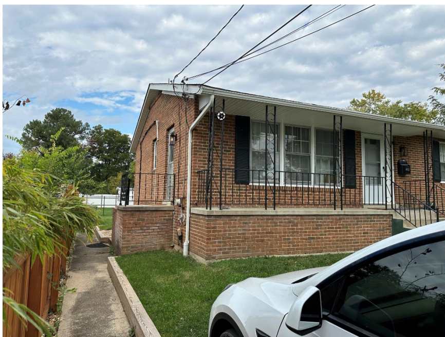
Figure 2: Southeast corner, 8002 54 th Avenue.
