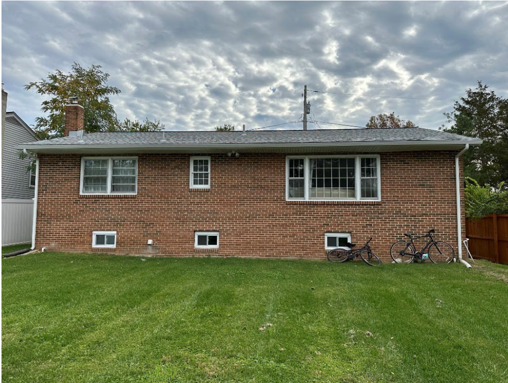
Figure 3: West (rear) elevation, 8002 54 th Avenue, October 2023.
