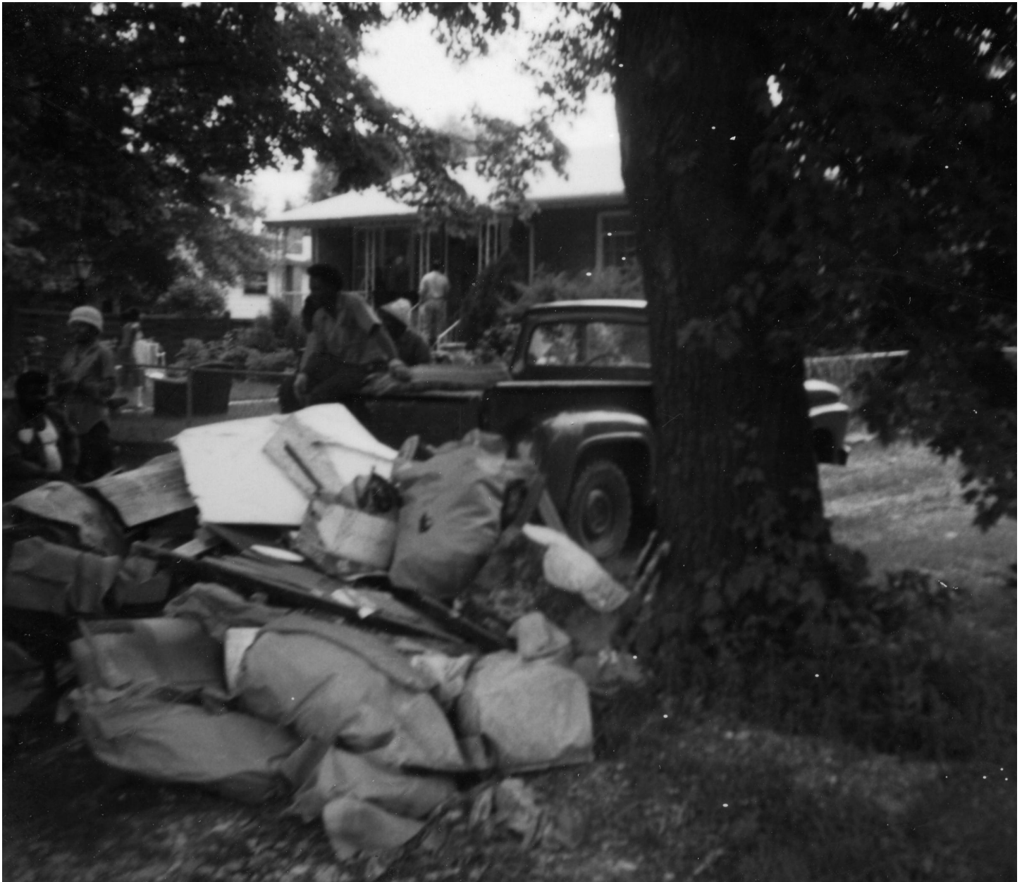
Figure 20: In 1972, Hurricane Agnes flooded the basement of the new home at 8002 54 th Avenue (in background). Lakeland Digital Archive.
