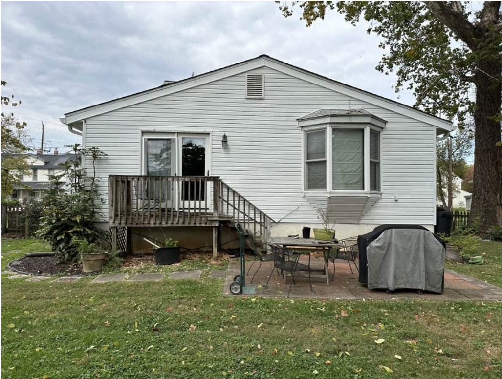
Figure 3. South elevation (rear), non-historic addition, 5011 Navahoe Street, November 2023
