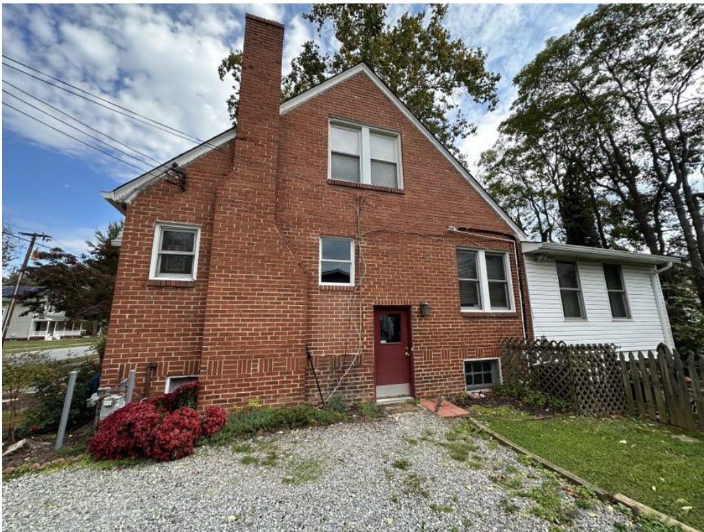
Figure 2. West elevation, 5011 Navahoe Street, November 2023
