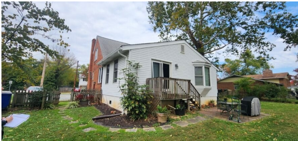
Figure 4. Southwest elevation, 5011 Navahoe Street, November 2023
