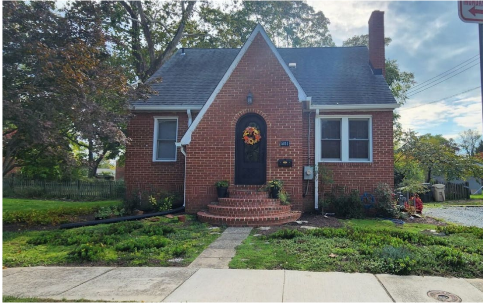
Figure 1: North elevation (façade), 5011 Navahoe Street
