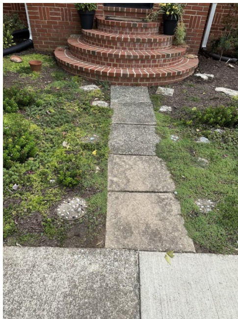
Figure 8: Concrete walkway leading to entrance staircase, 5011 Navahoe Street
