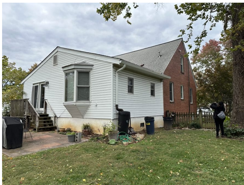
Figure 6: Southeast elevation, 5011 Navahoe Street
