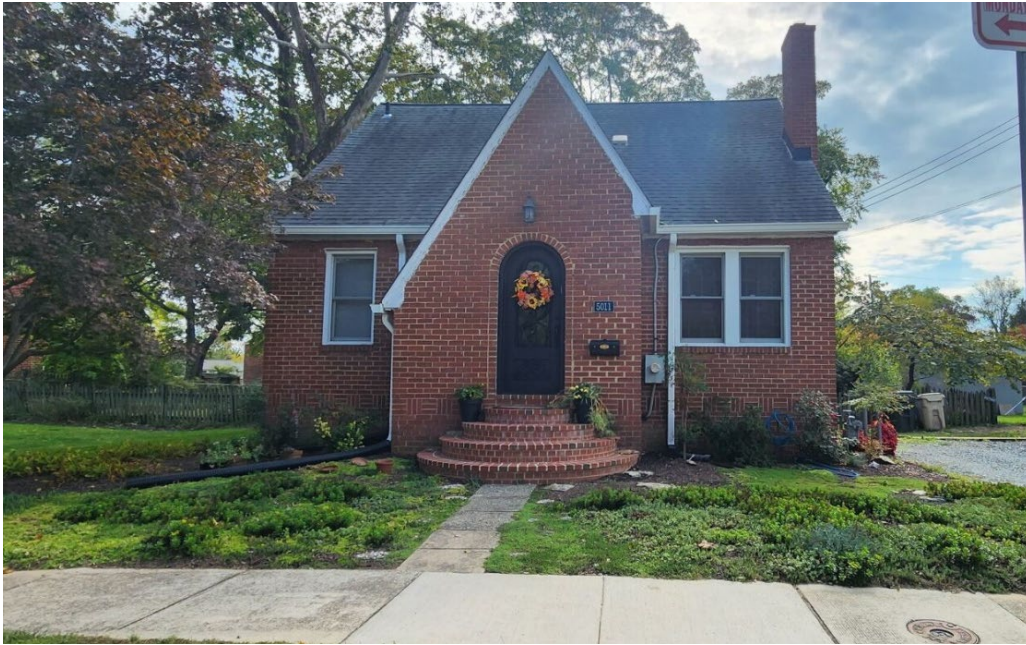
Figure 1. North elevation (façade), 5011 Navahoe Street, November 2023
