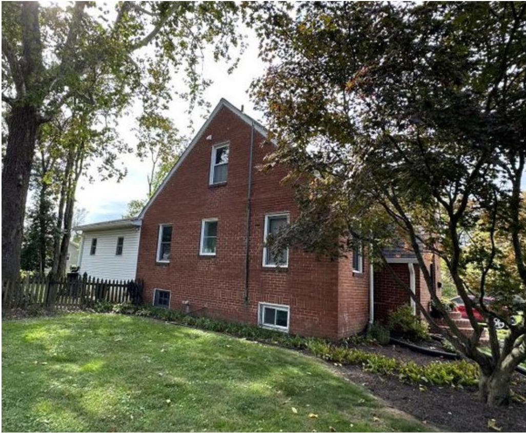
Figure 5. East elevation, 5011 Navahoe Street, November 2023
