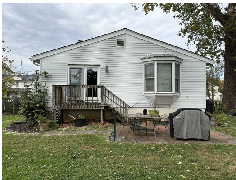
Figure 3: South elevation (rear), non-historic addition, 5011 Navahoe Street
