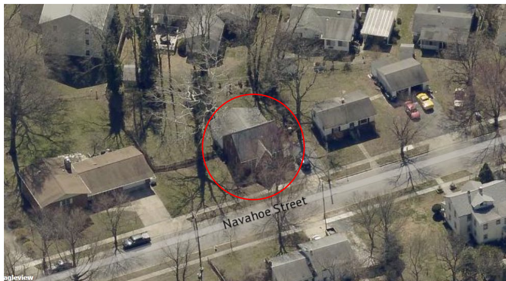
Figure 6. Nancy Tabbs House, oblique aerial view from north, December 2021. Source: Pictometry via PGAtlas.com.
