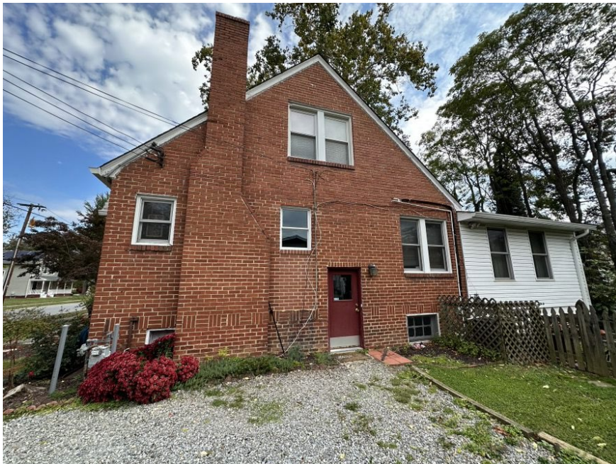
Figure 2: West elevation, 5011 Navahoe Street
