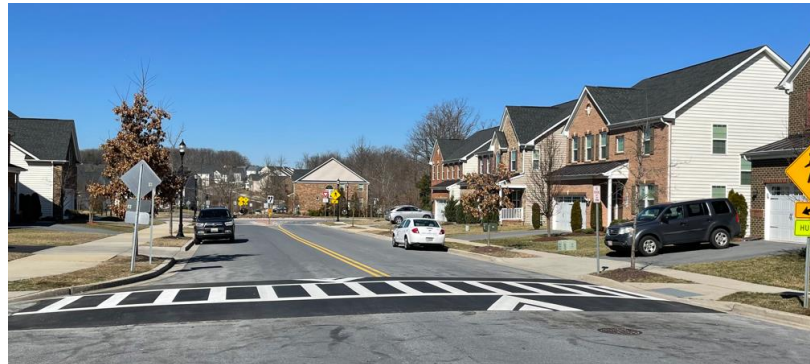
Raised Crosswalk – Level II
