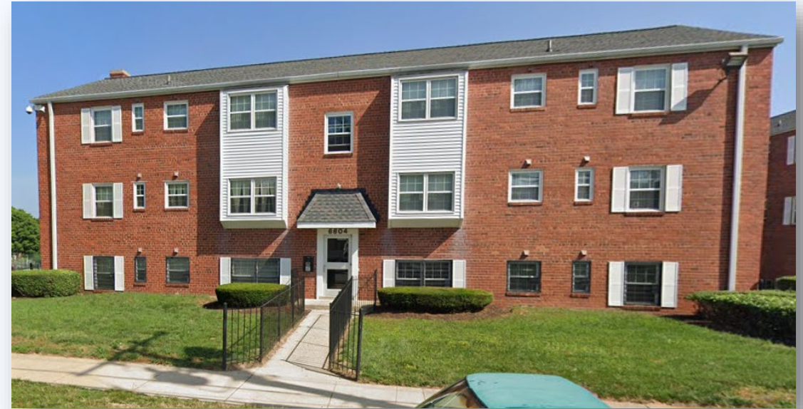
Pleasant Homes Apartments – 214 units preserved
