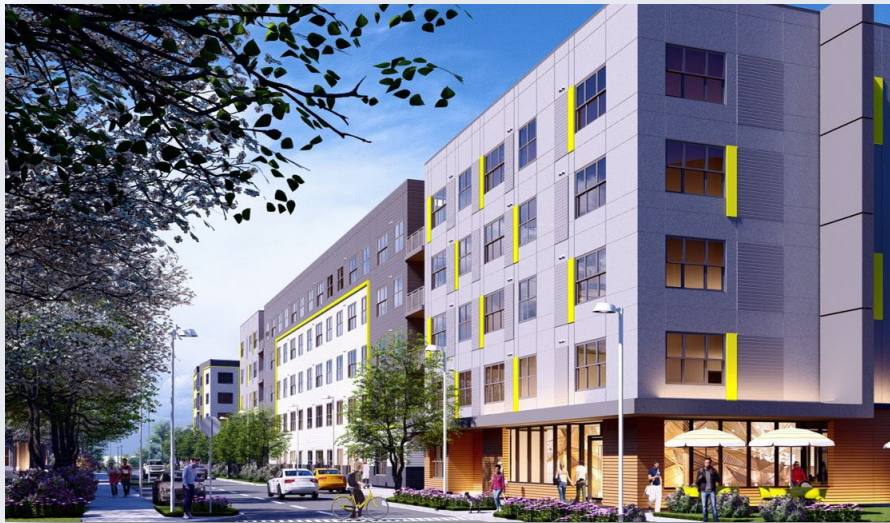
Sovren West Hyattsville Metro 147 units currently under construction Completion expected in 2024
