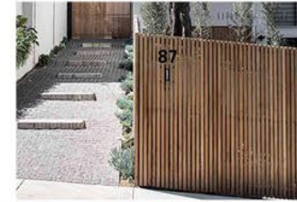
A Wood Slat Screen Wall
