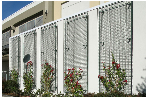
METAL PANELS ATTACHED TO FACADE
