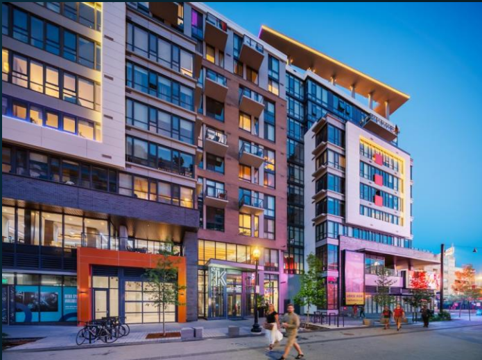
The Kelvin Mixed Use Development Project – NE DC.
