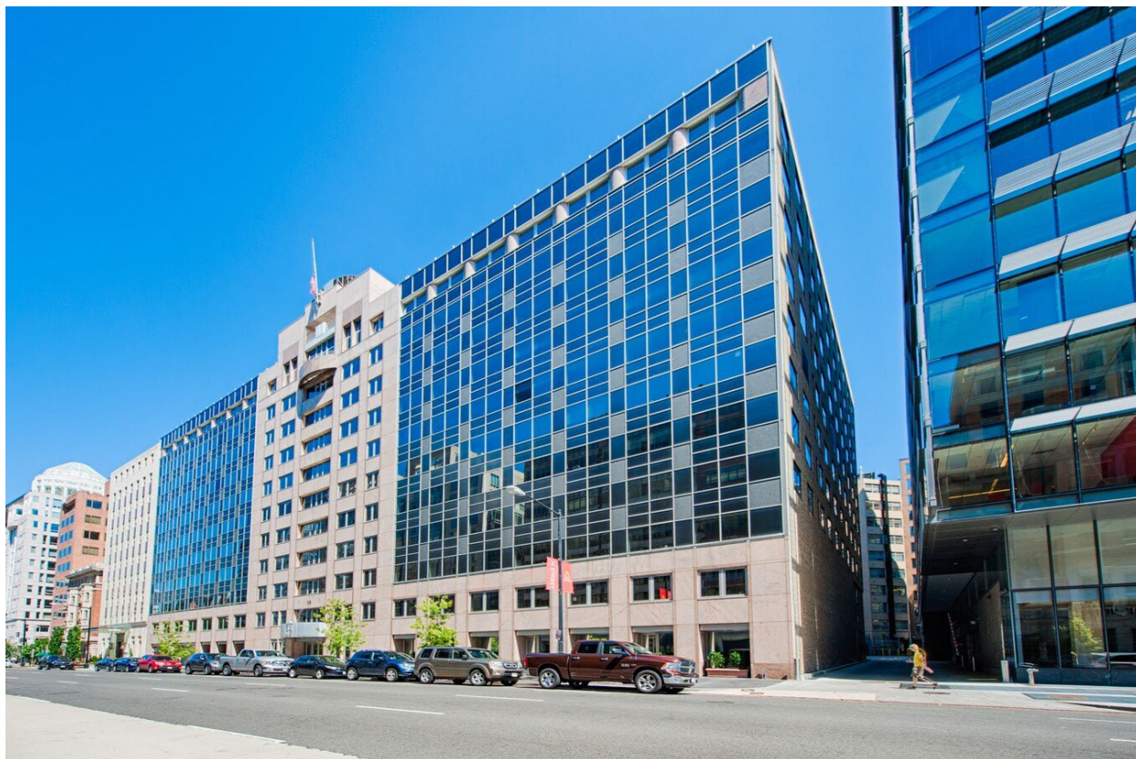
Figure 9: Matomic Building, 1717 H St. NW, Washington, D.C.
