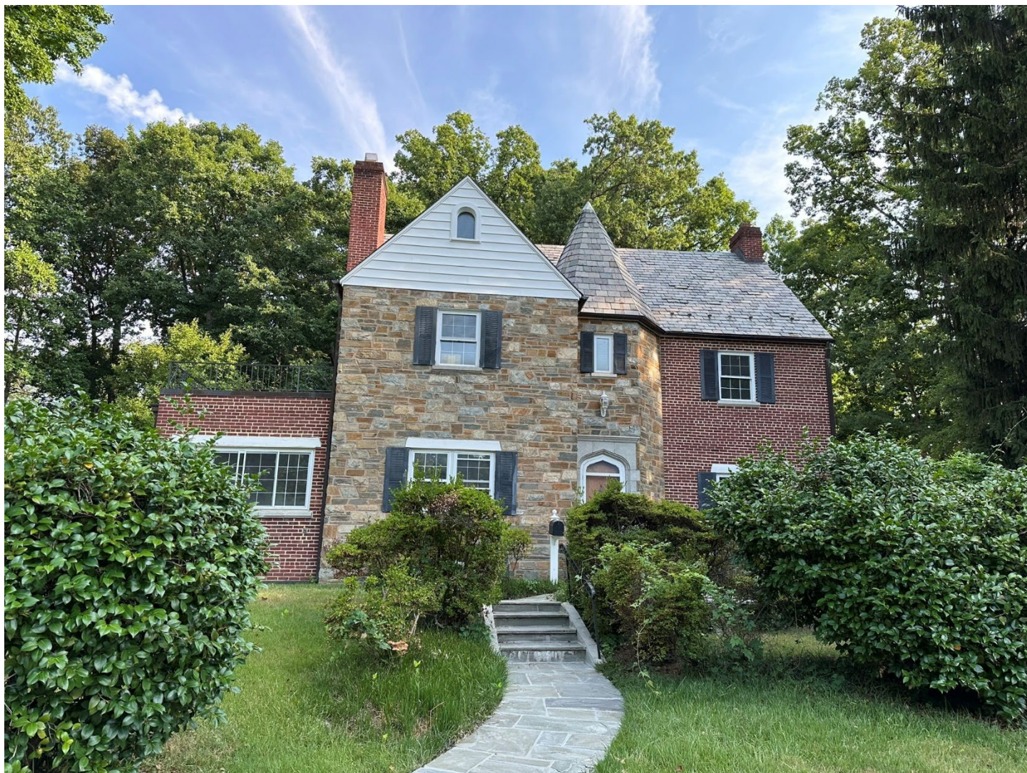
Maiatico House, south elevation, July 9, 2024.
