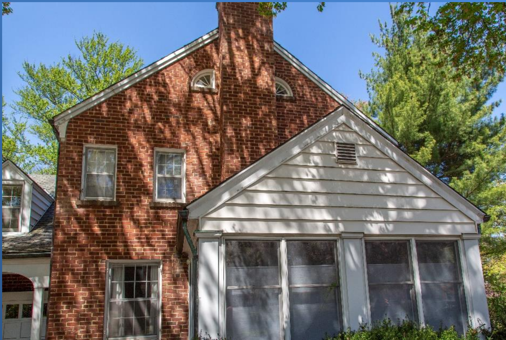
Yates and Mary Boswell House, south elevation, April 2023.
