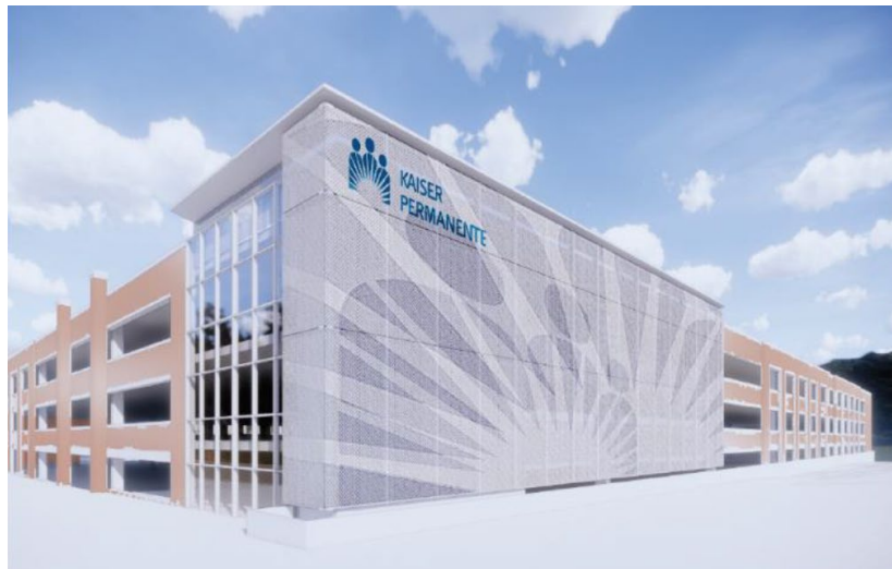
Art wall along the western façade of the parking garage.
