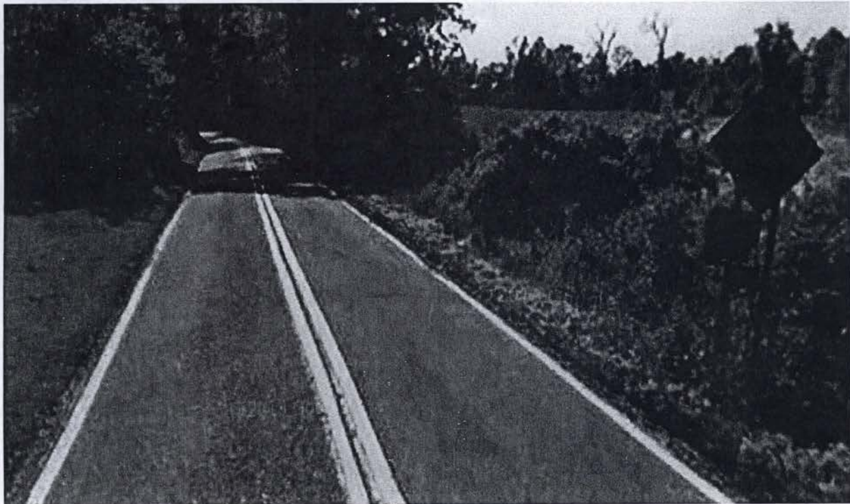
(approximately 16700 Queen Anne Bridge Road)
