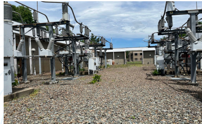
Central Ave Water Pumping Station Electrical Equipment and Switchyard Replacement
