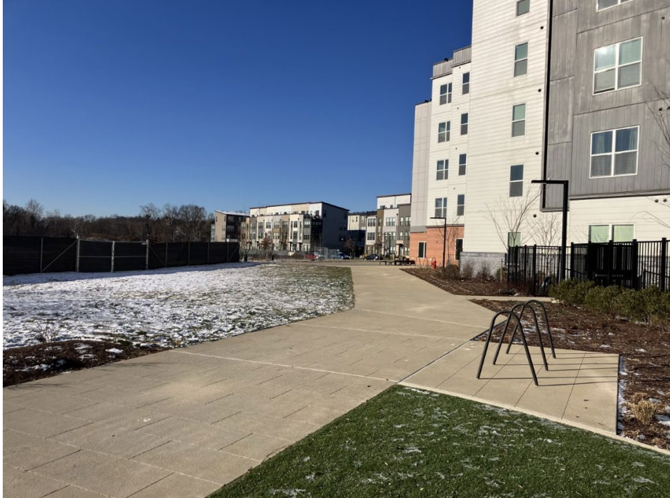
EXISTING PEDESTRIAN PROMENADE
