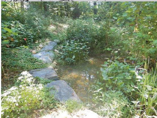
Precedent image of herbaceous buffering for root stabilization along eroded stream reaches.
