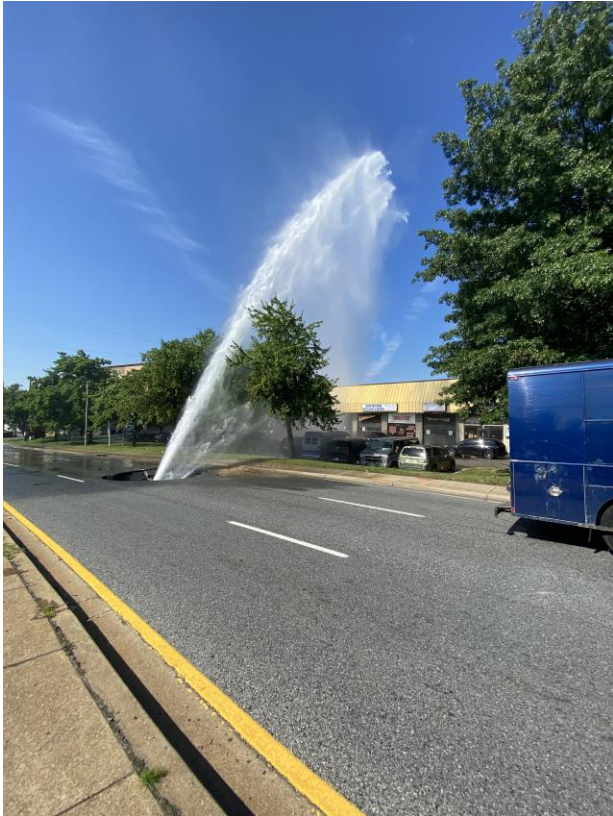
Capitol Heights Water Main Break July 2022
