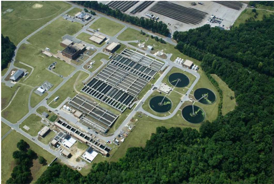
WESTERN BRANCH WRRF 30 MGD Upper Marlboro, MD
